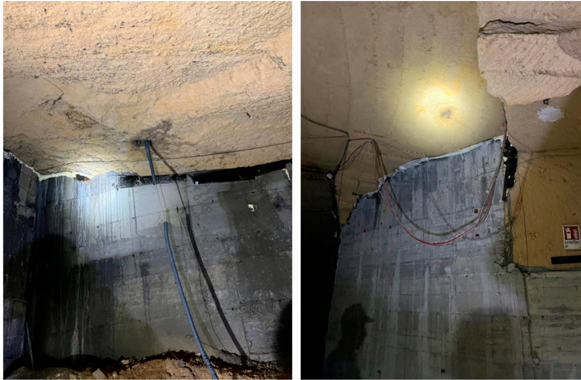
Figure 25. Photos of the consolidation interventions.
