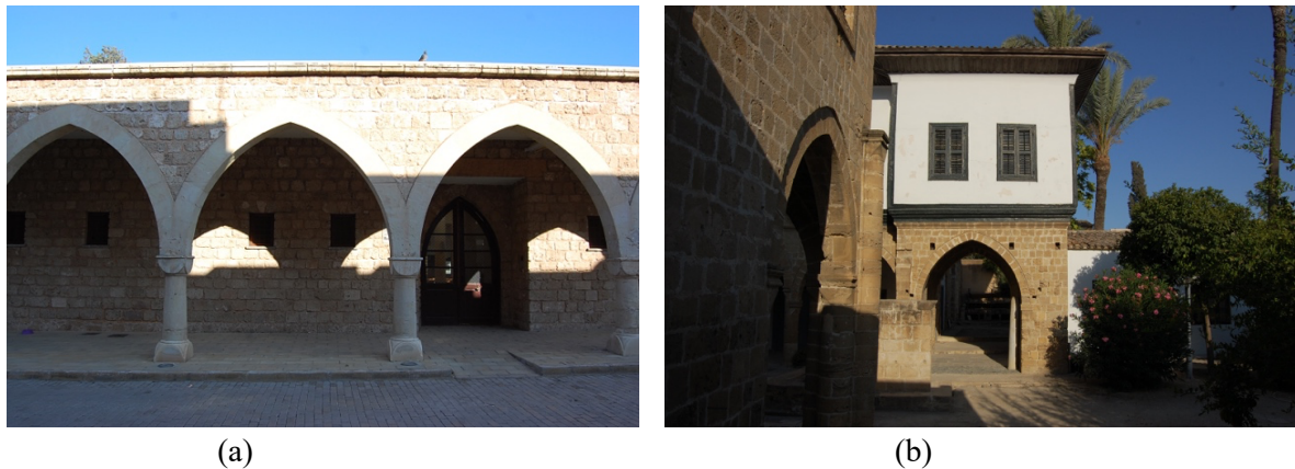
Fig. 9. (a) The arcaded colonnades are a transitional space that generates ventilation between the indoor spaces and the courtyard; (b) malqaf element for passive cooling in a vernacular house in Cyprus. Images Credit: Ozarisoy, (2023).
