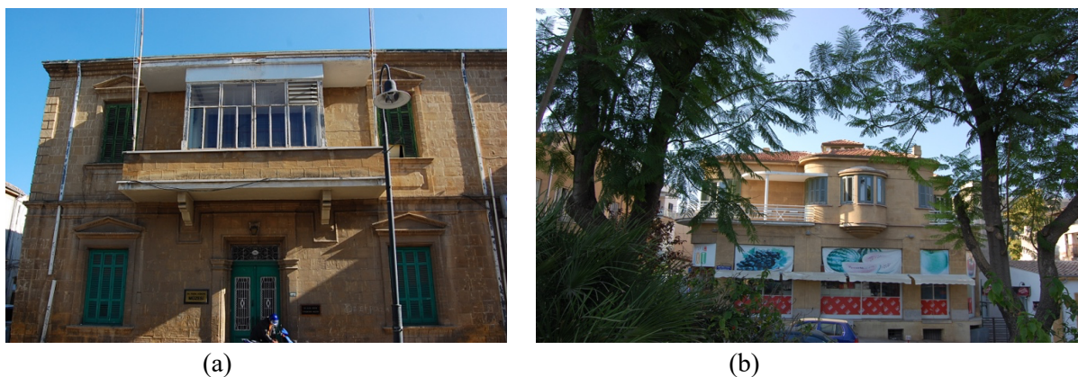
Fig. 8. (a) Elevation of the sunken room of a modern villa, which illustrates the use of mashrabiya, a design that incorporates a complete climatic system, including malqaf (b) Malqaf element for passive-cooling in a vernacular house in Cyprus.
