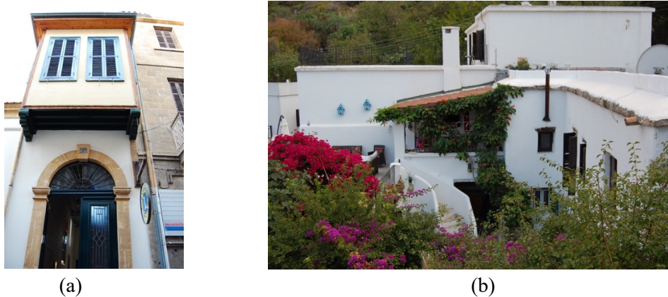
Fig. 10. (a) Overhang balcony space projection that shows ventilation generated by wind escape; (b) wind-catcher system in a vernacular house in Cyprus.
