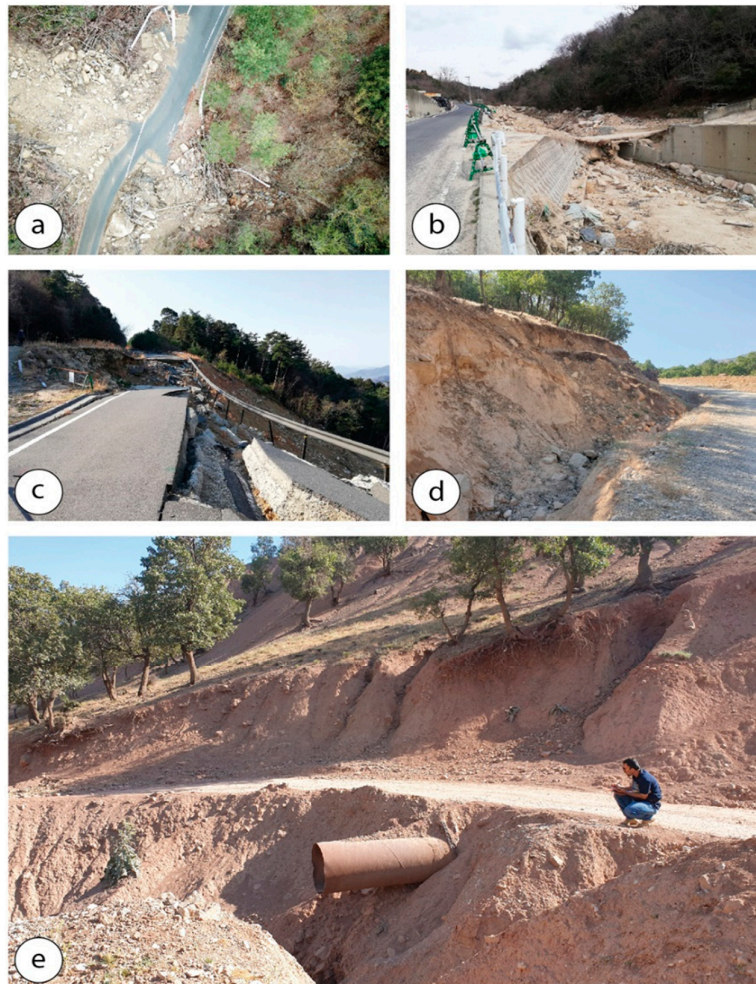
Figure 1. Road-side erosion from sudden and progressive events (a) Debris-flow apron in the mountain between Hiroshima City and Kure City in Japan after the 2018 heavy-rain event; (b) waterway erosion in near Kure City in Japan; (c) road collapse at the head-scarp of a landslide; (d and e) progressive road-side erosion and storm-water pipe erosion in Iran.
