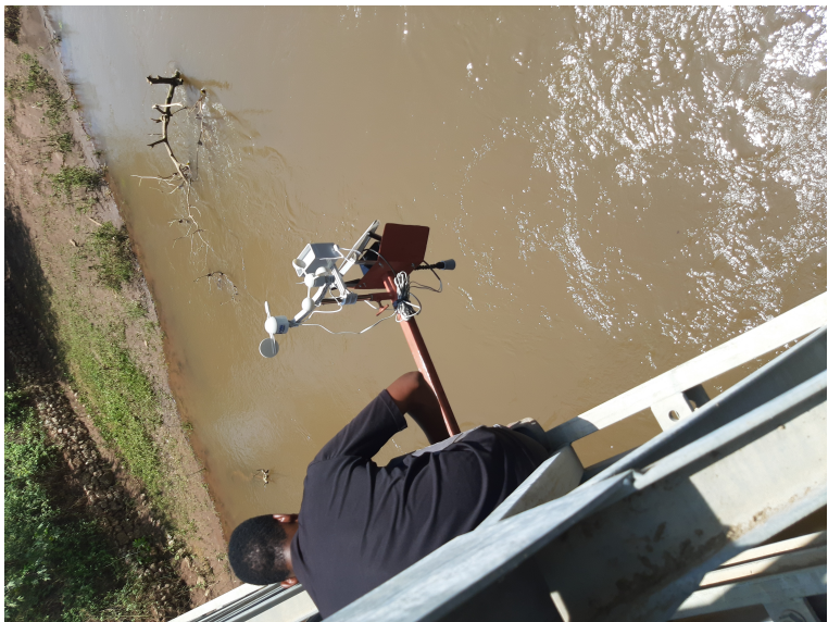
Figure 3. Sensor installation at Kikuletwa bridge
