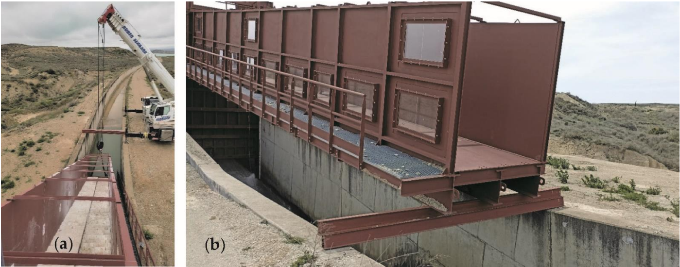
Figure 8. (a) Picture of the crane lifting the test chute. (b) Picture of the testing chute once lifted.
