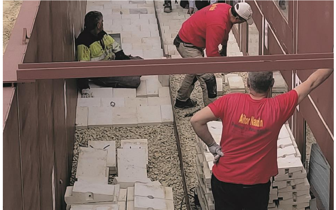
Figure 9. Picture of the placement of the WSB on the gravel bedding layer.
