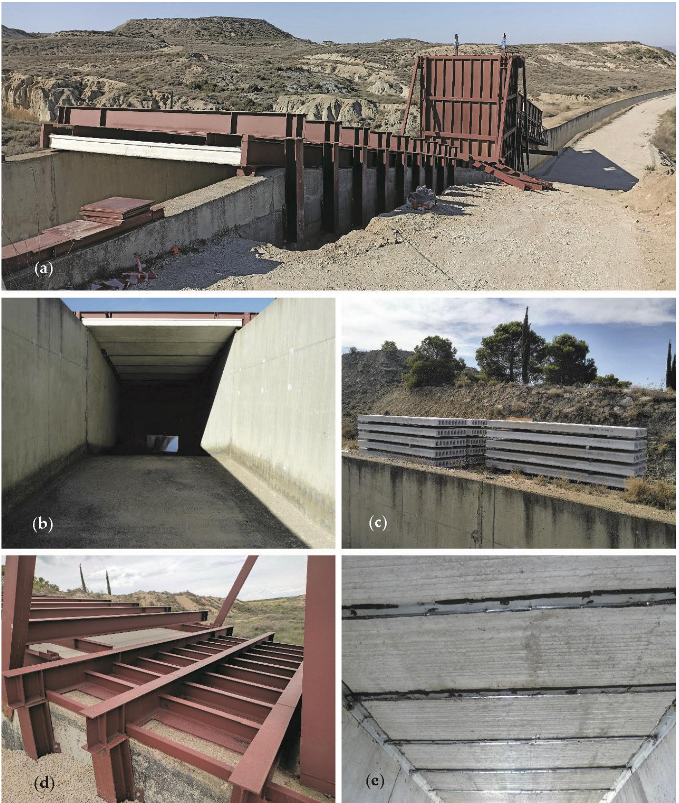
Figure 4. (a) View of HEFLR from the right bank of the auxiliary channel. (b) View of the interior of the auxiliary channel from upstream of the pressure channel. (c) Storage of the alveolar slabs used to cover the pressure channel. (d) Metallic frames used to support the alveolar slabs of the pressure channel and the metallic plates on the connection to the tower supply. (e) Detail of the sealing between the alveolar slabs and between the slabs and the channel walls (view from inside the pressure channel).
