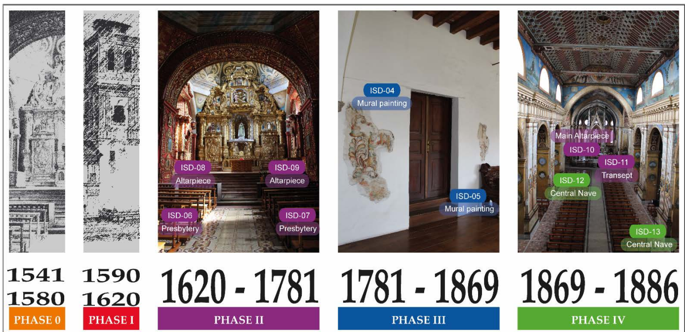
Figure 2. Image of the five chronological phases of the construction of the Santo Domingo church in 345 years. (1541-1580) Earth construction; (1590-1620) Phase I; (1620-1781) Photography of the Chapel of the Rosary; (1781-1869) Photography of the mural in the convent corridor; and (1869-1886) Photography from the central nave to the main altar, with the location of the places where the mortar samples were extracted.
