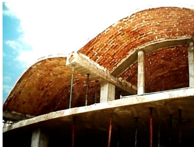
Figure 3. Vault pieces constructed in hollow thin brick by the authors in Seville
