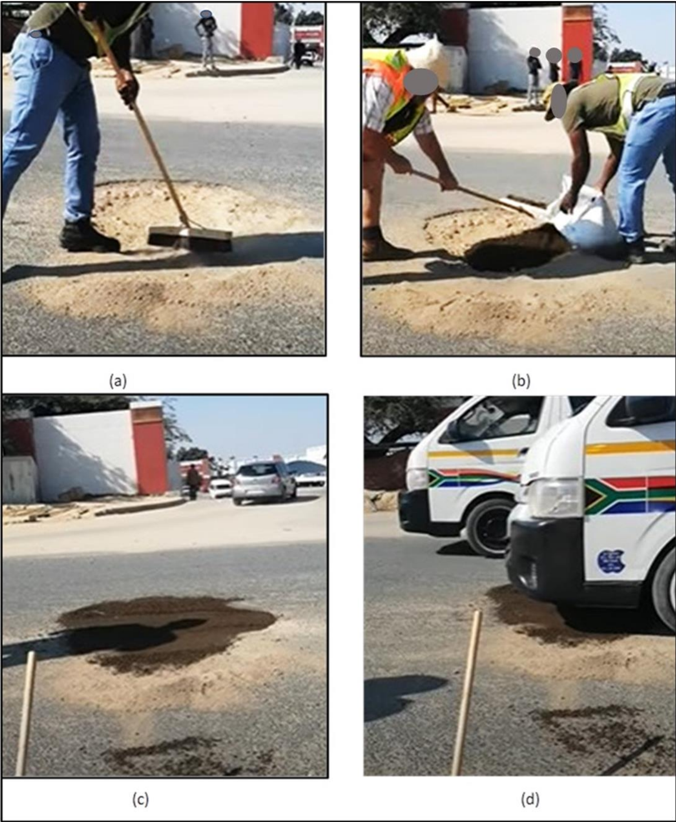
Figure 12: (a) Cleaning of pothole; (b) filling pothole with a water-resistant anionic NME gravel [23] (refer Acknowledgements); (c) hot-hole filled and partially compacted by hand, and (d) vehicles driving over filled pothole and increase compaction.
