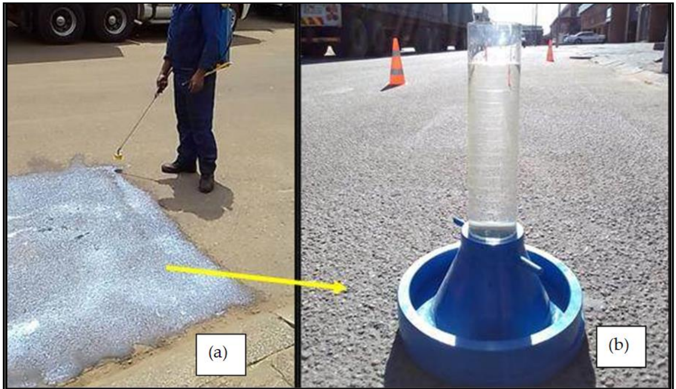
Figure 5: (a) Application of a clear-seal by hand-sprayer at a rate of approximately 1 to 2 l/m 2 (about 5 to 10 ml of NPNS /m 2 at a material cost of about US$ 0.10 to US 0.20 /m 2 ) – note the close proximity of the sprayer head to the road surface to prevent loss during windy conditions; (b) the dried surfacing 30 minutes after application of the clear-seal with a Marvil apparatus placed on top of the surfacing to measure the rate of water penetration into the treated surface.
