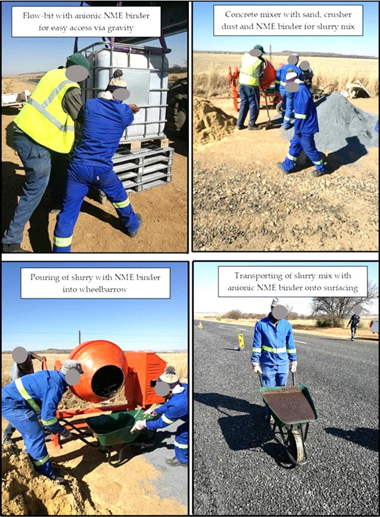
Figure 16: Labour-intensive road-side manufacturing of the slurry mix for an anionic NME binder slurry seal or for a modified Cape seal using an anionic NME binder.
