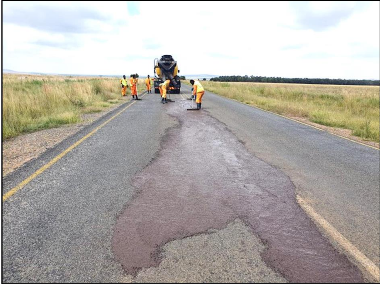
Figure 18: Filling of deformed areas on the road surface using a medium NME slurry mix as a pre-treatment to address severe deformation before applying a NME slurry across the whole width of the lane and road as shown in Figures 14 and 15.
