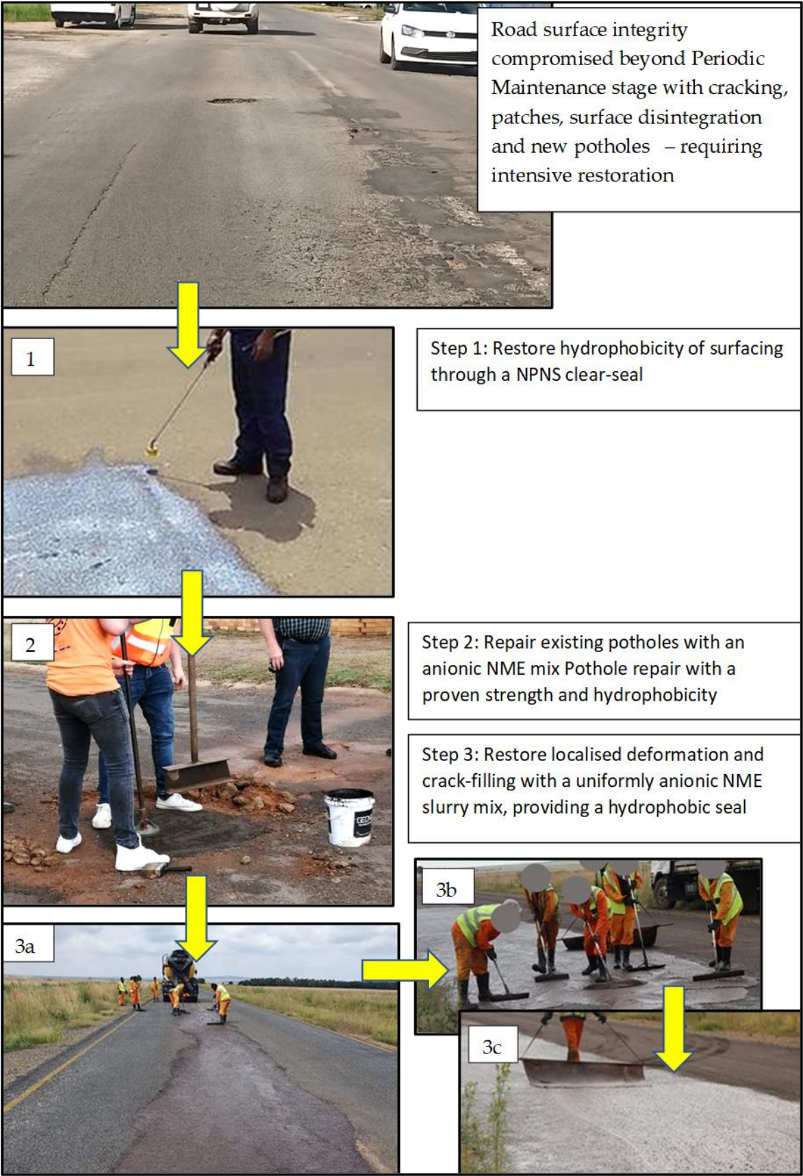
Figure 19: Recommended restoration of compromised road surfacings using available proven nanotechnology solutions suitable for labour-intensive application for rapid job creation providing valuable asset protection.
