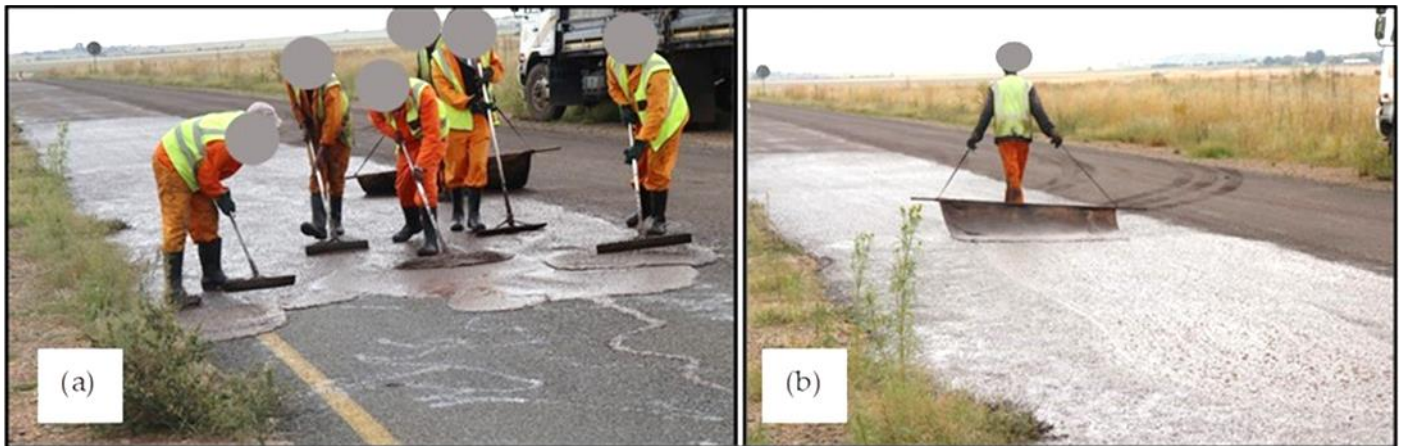
Figure 14: Application of a labour-intensive anionic NME slurry seal to effectively provide a water-repellent new surfacing, preventing water-ingress into the pavement structure on a severely cracked surfacing without disturbing the existing surfacing and restoring some riding quality – this surfacing will dry within 6 hours due to the water-repellent addition of the nano-silane – the anionic NME modified binder slurry seal is mixed to provide a six hour working envelope, found to be practical on actual projects, while creating a permanent bonding to the old surfacing and a water-resistant surfacing.
