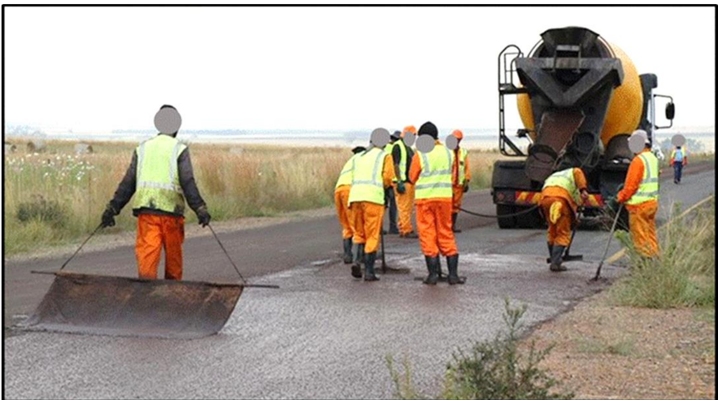
Figure 15: Slurry NME mix supplied to site using a large concrete mixer - spread using hand operated squeegees and obtaining the required texture with a hessian-mat dragged by hand.
