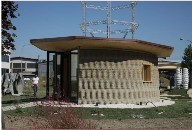
Figure S1. The Gaia House by WASP: first prototype of a 3D printed earthen building, with biodegradable materials (built in 2018) [source WASP].
