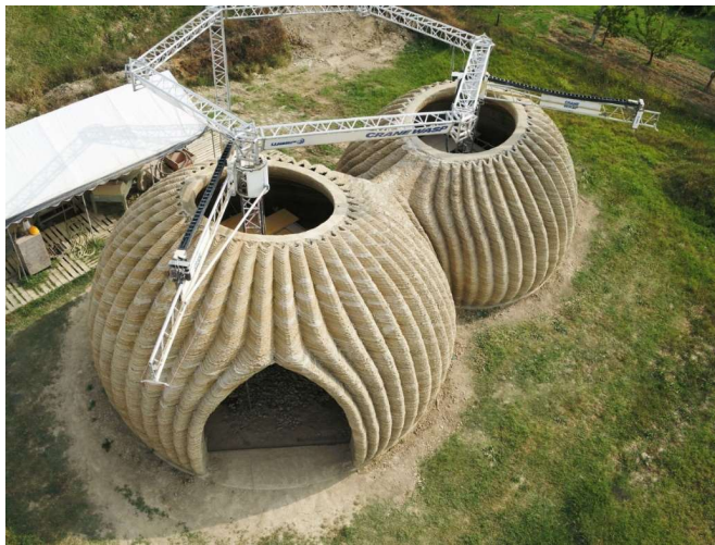
Figure S2. The Tecla House by WASP: 3D printing of the second prototype of an earthen building (completed in 2021) [source WASP].
