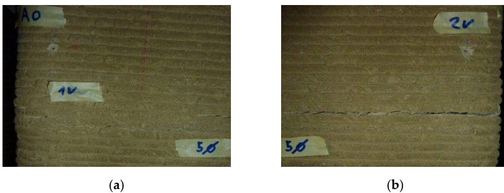
Figure 10. Details of the detachments between the horizontal layers of the side to the left of the operator: (a) Left detachment, which reaches edge 1; (b) Right detachment, which reaches edge 2.
