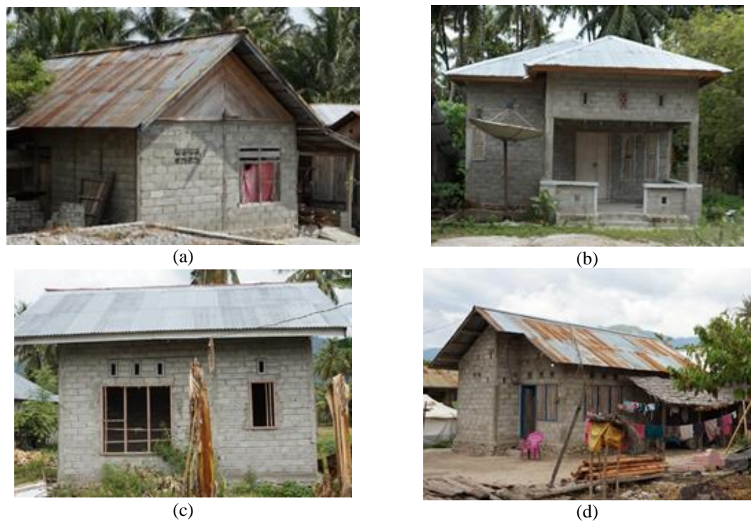
Figure 2. Examples of poorly built houses from the Palu (Central Sulawesi) Earthquake on September 28th, 2018
