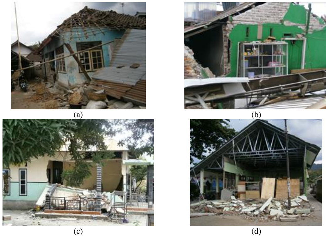
Figure 4. Examples of poorly built houses from the Lombok Earthquake on July 29th, 2018
