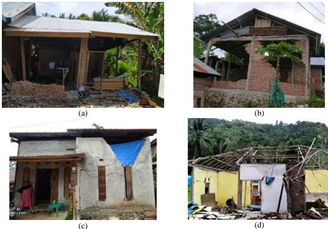
Figure 1. Examples of poorly built houses from the West Sulawesi Earthquake on January 15th, 2021
