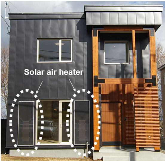
Figure 5. Facade of the house with the solar air heater on external wall.
