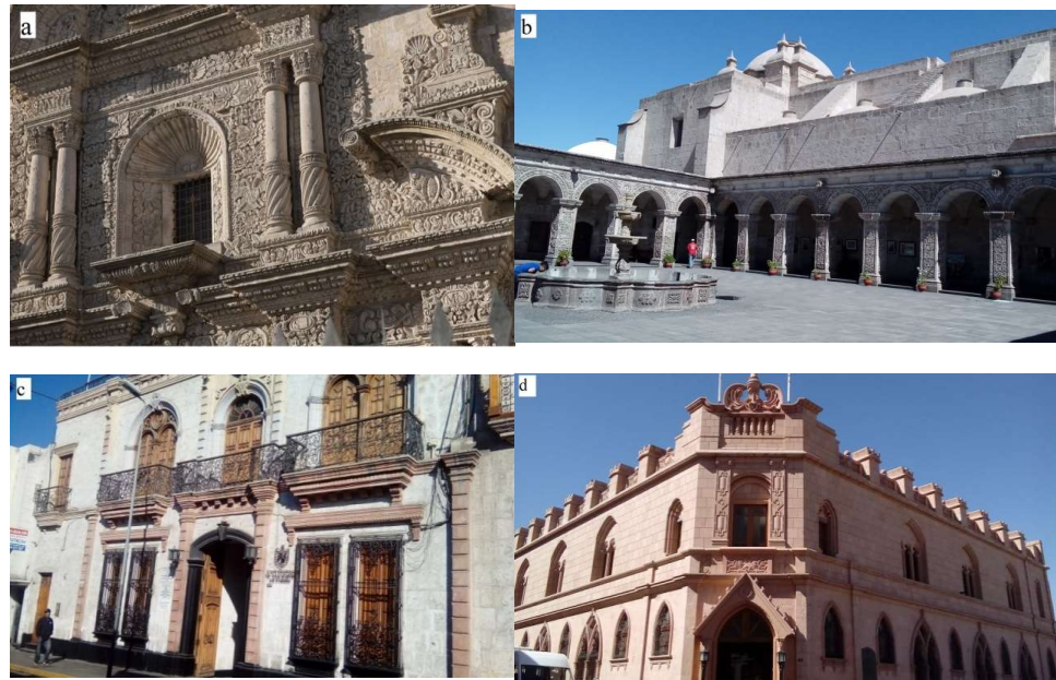
Figure 1. (a) Carved white ignimbrite façade of La Compañía de Jesús church, ca. 1698; (b) Restored cloister after 1960 earthquake; (c) Pink ignimbrite pilasters, corbels and moldings; (d) Neogothic Bishop's Palace (the latter two from the first quarter of the 20th century)
