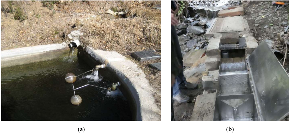
Figure 14. Installed mechanisms which regulate water extraction (a) and distribution boxes (b) restricting the amount of legally allowed water for exploitation.
