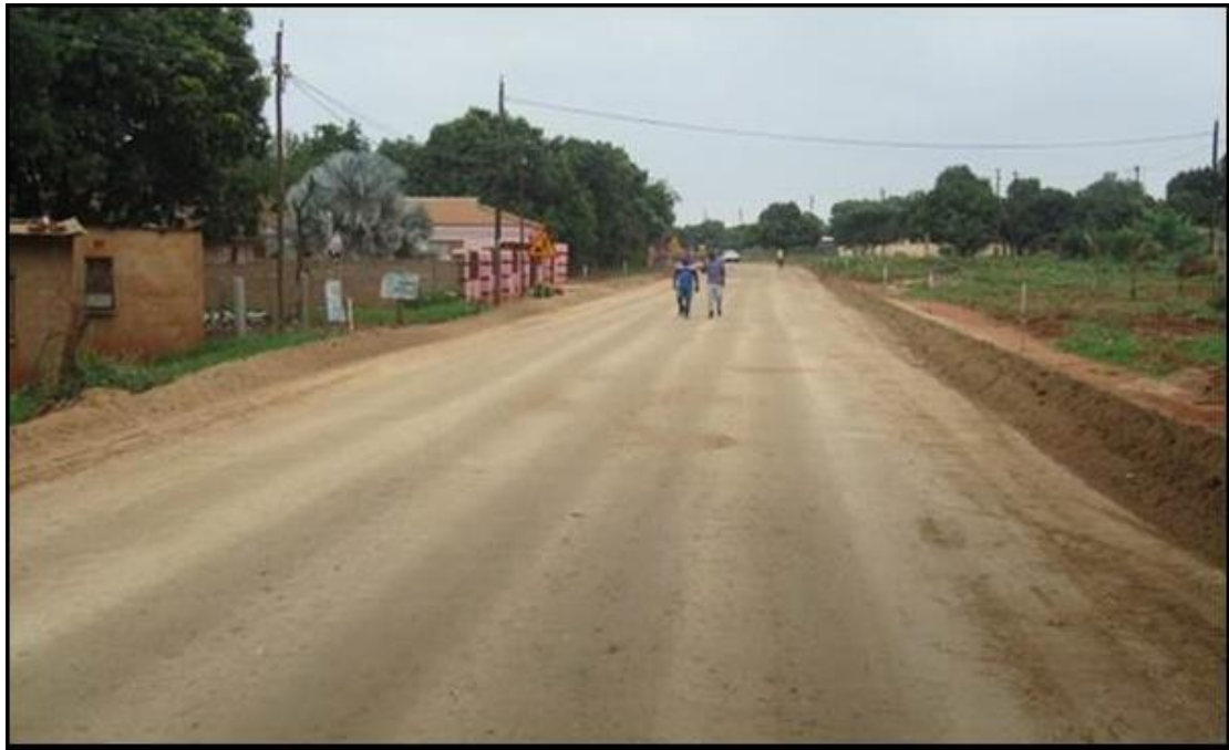
Figure 12: Recycled road with NME stabilisation opened to local traffic to provide access to houses – with no protective prime or surfacing added (note the same pink painted façade of the same house shown in Figure 11(a))
