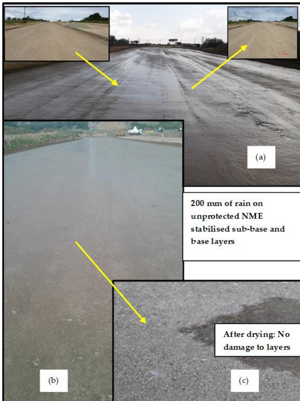
Figure 9: One week after placement of base (1.2% NME – 0.7% residual bitumen) and the exposed sub-base (0.7% NME – 0.4% residual bitumen) – 200 mm of rain fell with (a) the sub-base layer, and (b) base layer representing rivers; (c) after drying no water related damage could be observed
