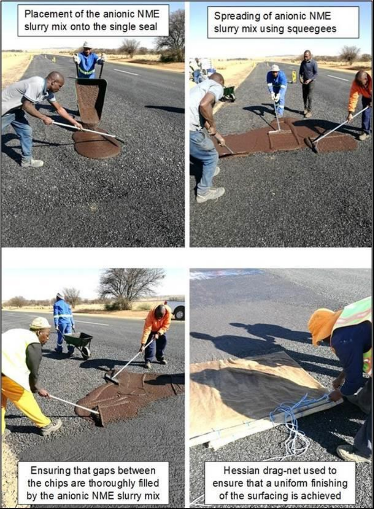
Figure 20: Labour-intensive construction of a modified Cape seal using an anionic NME binder with the slurry mixed on site next to the road
