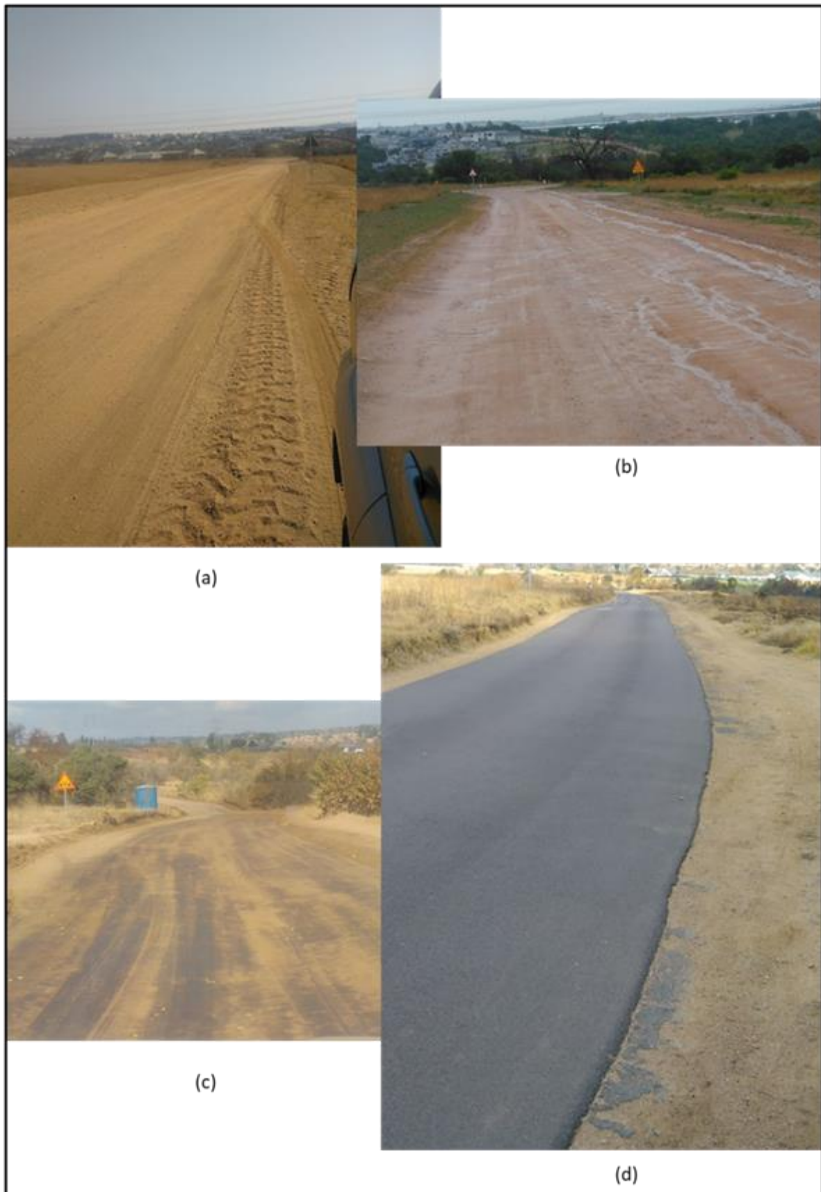
Figure 21: Upgrading of a local access road with (a) and (b) showing the sandy/slippy/muddy conditions prior to upgrading; (c) 100 mm in-situ stabilisation with an anionic NME stabilising agent and (d) with an ultra-thin fine-graded asphalt surfacing (specified by client)
