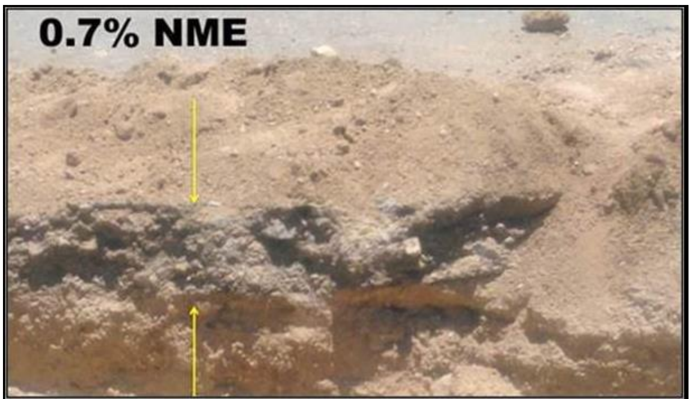
Figure 16: Cut through the stabilised sub-base constructed using a water-cart for distribution of the 0.7% anionic NME stabilising agent added to the construction water, mixed by grader and compacted
