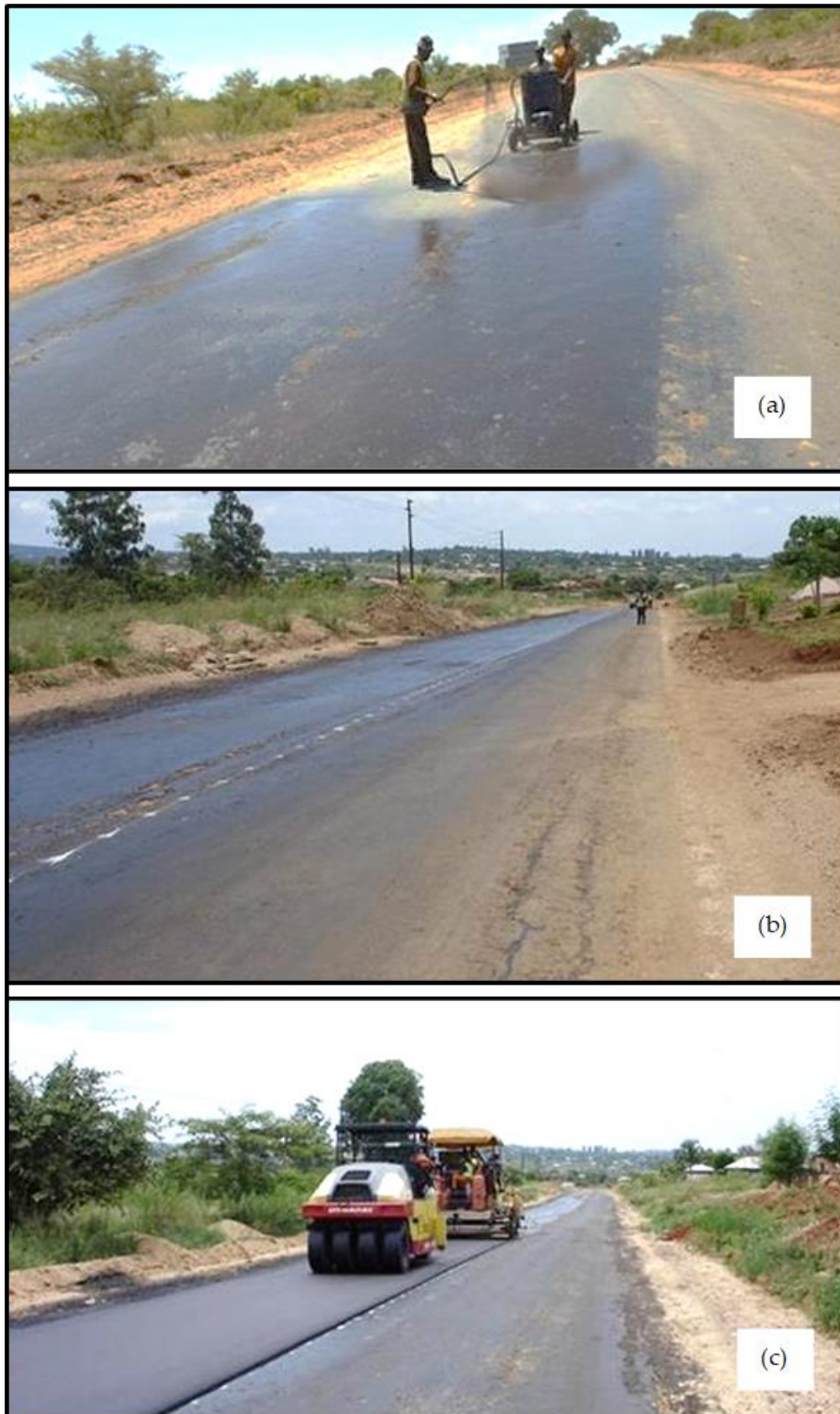
Figure 13: (a) Hand application of a quick drying anionic diluted NME prime coat to protect the base before application of the surfacing; (b) applying of a tack coat 2 months after construction of the base layer (opened to traffic); (c) applying of the surfacing – note the little damage to the base layer after two months open to traffic during the holiday and rainy season
