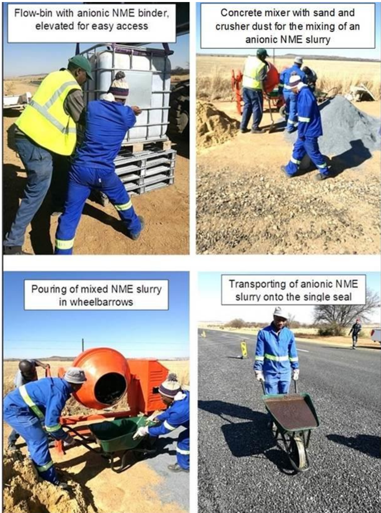
Figure 19: Labour-intensive road-side manufacturing of the slurry mix for a modified Cape seal using an anionic NME binder
