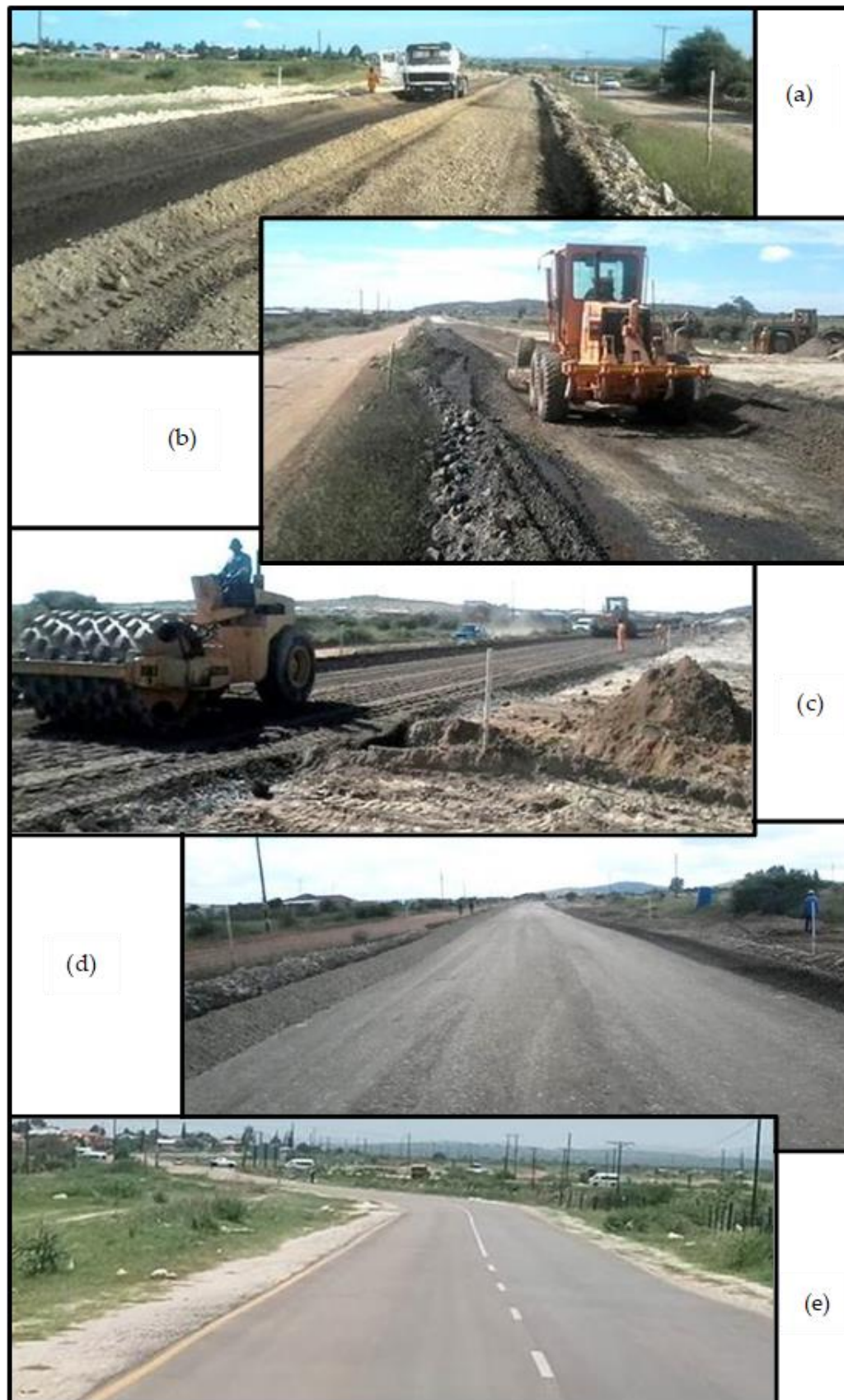
Figure 17: (a) Water-bowser with construction water and anionic NME stabilising agent; (b) Single grader used for mixing of the anionic stabilising agent pre-mixed within the construction water; (c) Compaction and cutting of final layer levels; (d) Condition of the compacted layer prior to applying a tack-coat and surfacing; (e) Condition of the surfaced road 6 years after completion
