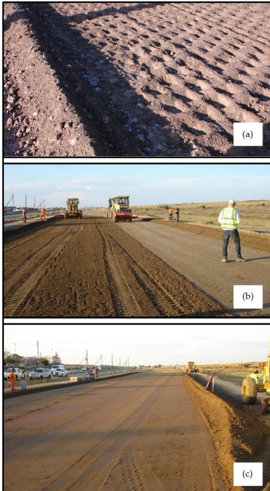
Figure 15: Compaction of the layer with the anionic NME mixed into the layer using conventional equipment; (a) using a sheep-feet roller; (b) followed by a vibratory steel-drum roller and a pneumatic roller to create a smooth surfacing; (c) a small percentage of the NME mix is retained in the tanker as an enrichment of the top of the layer before final compaction (note that similar to normal emulsion stabilisation, clean water should not be sprayed onto the layer)
