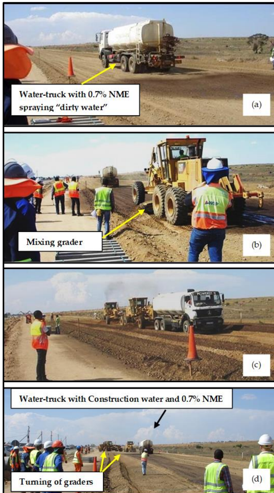
Figure 14: The sub-base granular material is spread along the section to be stabilised and compacted allowing for the compaction factor; (a) the water-bowser containing the anionic NME pre-mixed with the required construction water is starting with the spraying of the NME mix; (b & c) the water bowser is closely followed by graders that are mixing the NME stabilising agent dissolved in the construction water over the pre-determined length and width of the road to be stabilised; (d) due to the turning movements and continued process of spraying and mixing, the construction of a section of road using conventional equipment is considerably more time consuming compared to the use of central mixing plants with paving equipment or with recycling equipment
