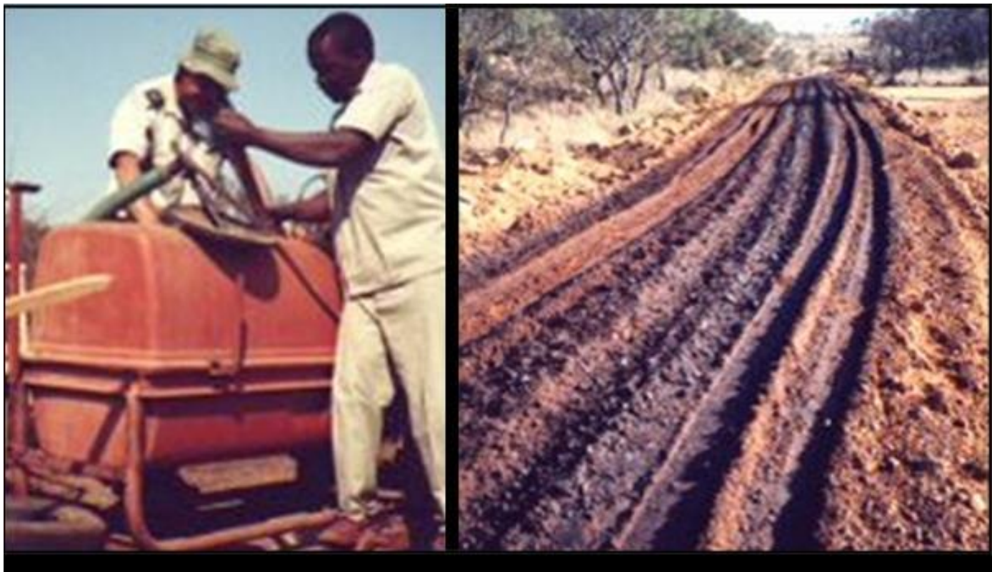
Figure 49: Addition of the material compatible anionic NME stabilising agent to a hand-operated sprayer and application of the anionic NME stabilising agent premixed with construction water on the ripped in-situ material
