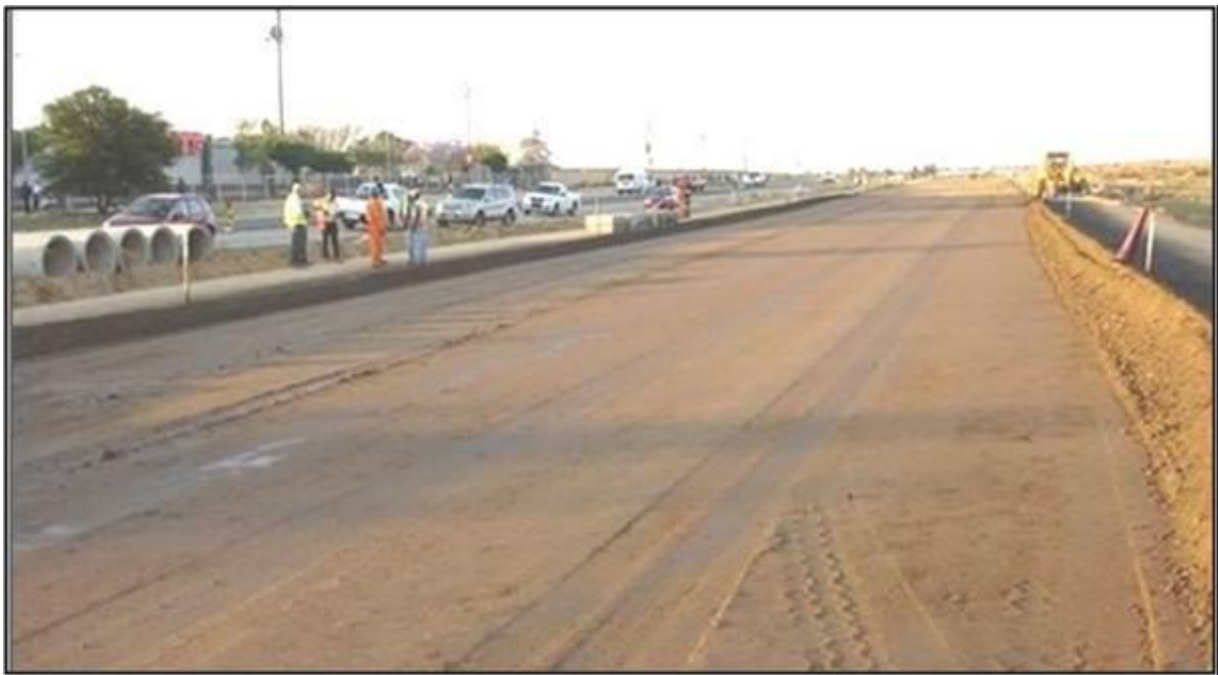
Figure 37: Enrichment of the top of the layer through spraying of the last of the diluted (with construction water) anionic NME stabilising agent before final compaction
