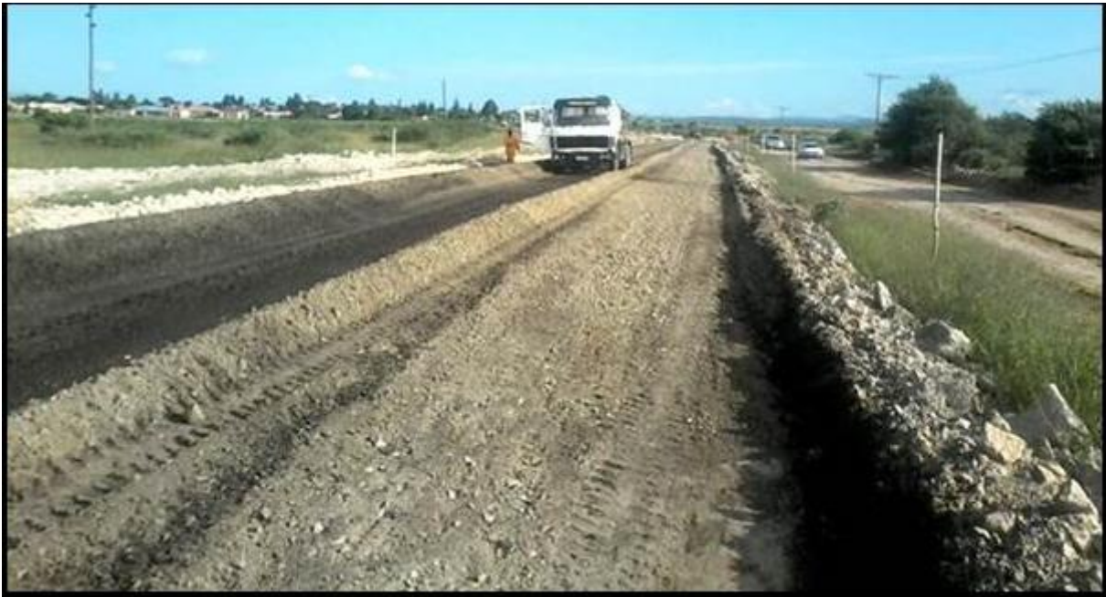
Figure 42: Water-bowser with construction water and anionic NME stabilising agent
