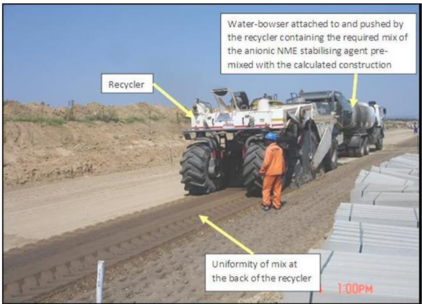
Figure 22: Mixing of the anionic stabilising agent using a recycler with a fitted micro-processor which controls the application of the NME stabilising agent pre-mixed with the construction water
