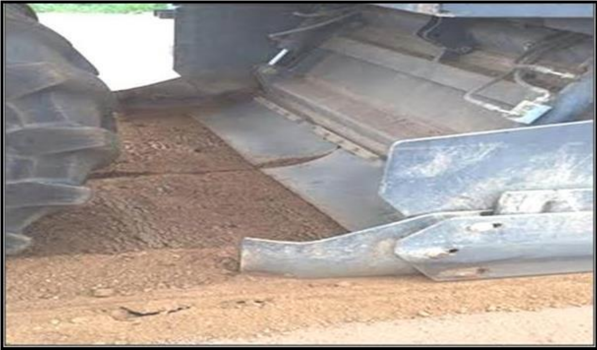
Figure 26: Material directly behind the recycler of the road shown in figure 25, with the NME stabilising agent, pre-mixed with the construction water, already added
