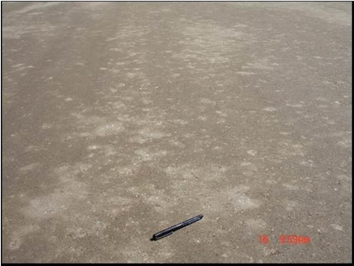
Figure 17: Placement of the 150 mm base layer by paver after compaction – note the texture of the finishing achieved
