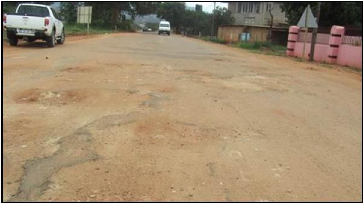
Figure 24: Typical condition of a severely distressed urban road with numerous pot-holes and materials not conforming to traditional standards for in-situ treatment using traditionally used stabilising agents
