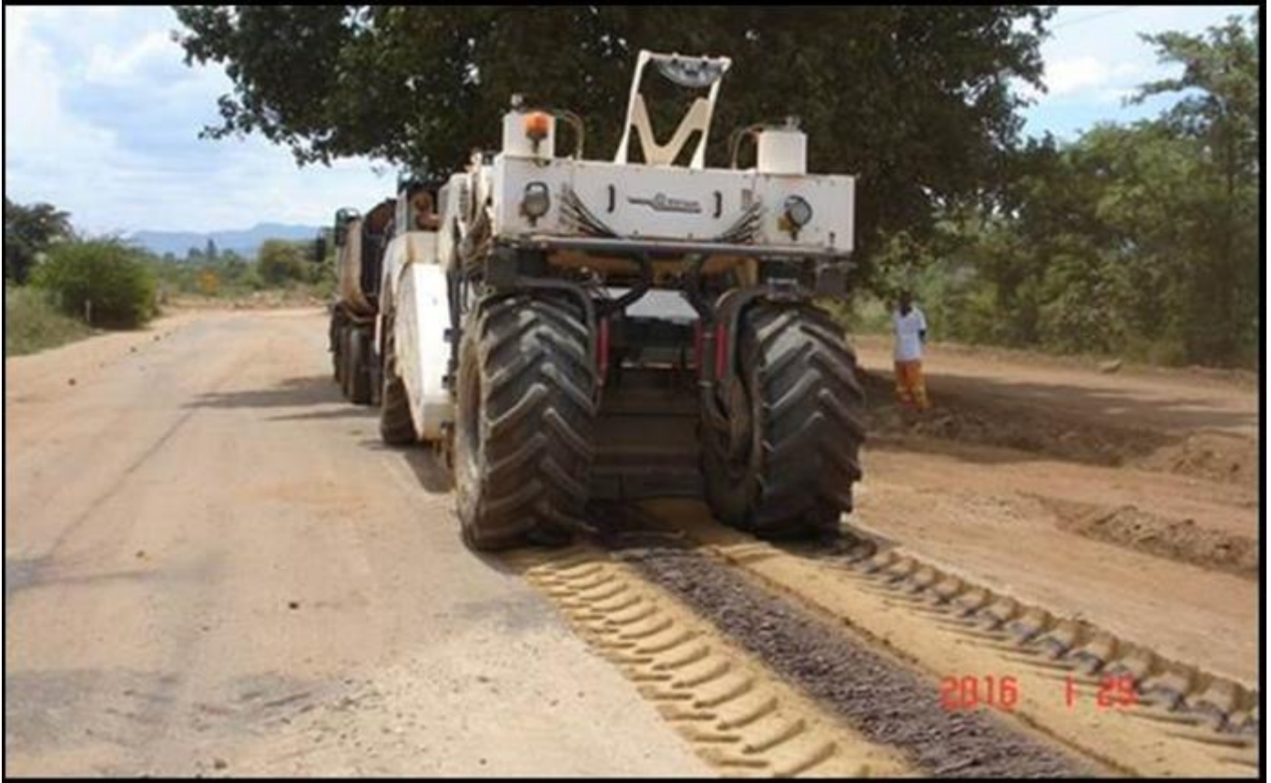
Figure 59: Uneven distribution of the stabilising agent behind the recycler caused by blocked spray-nozzles
