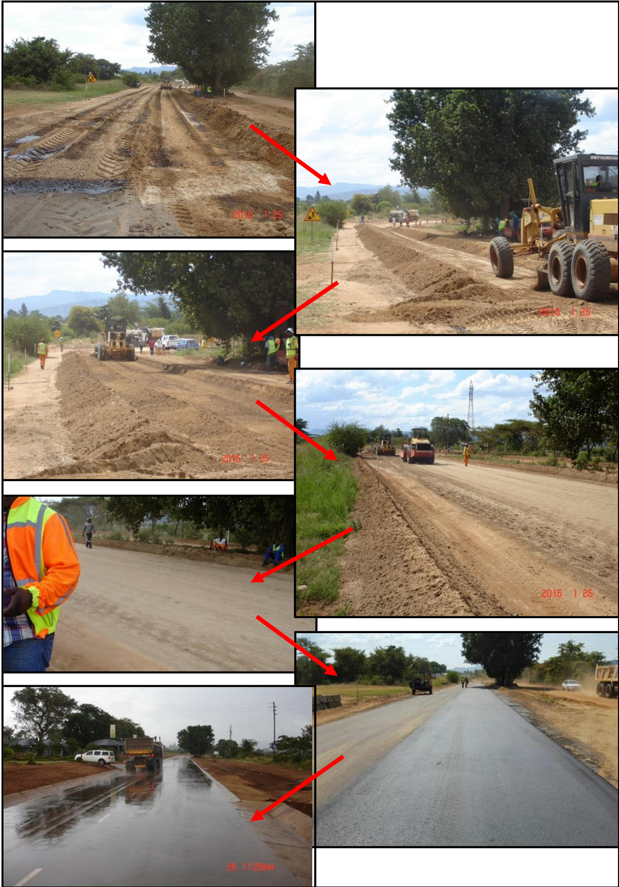
Figure 60: Resolving the uneven distribution of the NME stabilising agent trough the remixing of the road pavement layer using conventional equipment
