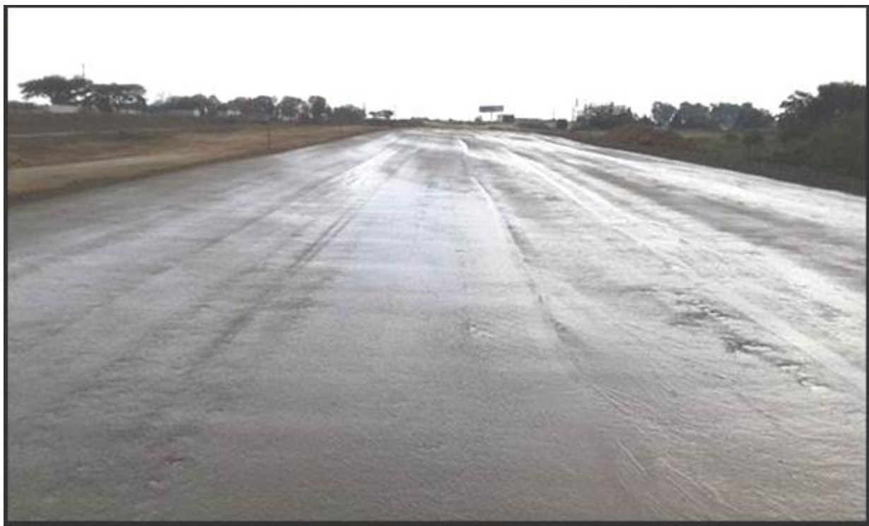
Figure 39: Similar to the exposed base layer (Figures 19 and 20), the sub-base was also subjected to 200 mm of rain in a single week soon after construction
