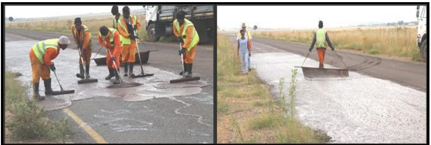
Figure 64: Application of a labour-intensive anionic NME slurry seal to effectively provide a water-repellent new surfacing, preventing water-ingress into the pavement structure on as severely cracked surfacing without disturbing the existing surfacing and restoring some riding quality – this surfacing will dry within 6 hours due to the water-repellent addition of the nano-silane – a six hour working envelope is created by dilution the anionic NME modified normal slurry mix by 50:50 with water, reducing the bitumen content by about 50% while creating a permanent bonding to the old surfacing and a water-resistant surfacing
