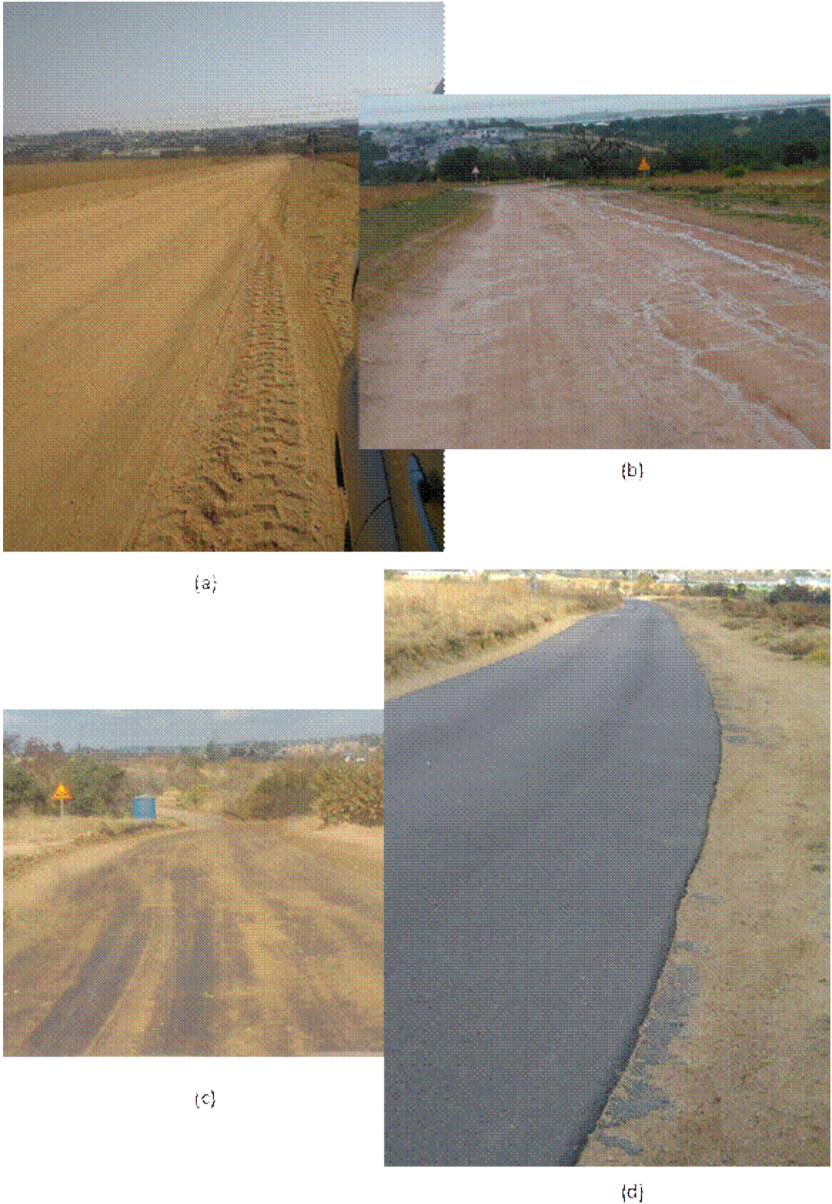
Figure 54: Upgrading of a local access road with (a) and (b) showing the sandy/slippy/muddy conditions prior to upgrading; (c) 100 mm in-situ stabilisation with an anionic NME stabilising agent and (d) with a ultra-thin fine0graded asphalt surfacing
