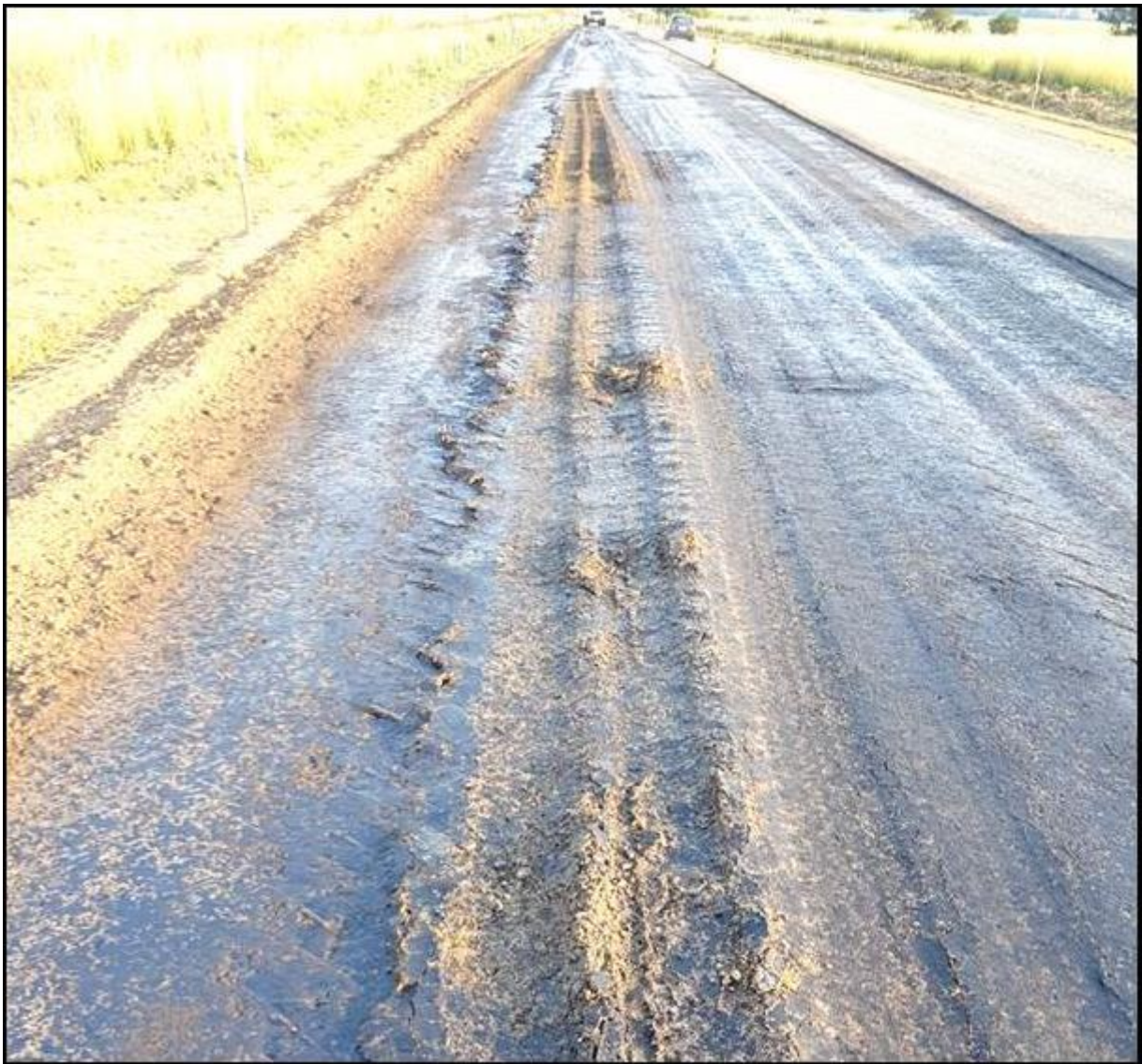
Figure 56: Severe movement of the NME stabilised layer indicative of layer thicknesses not complying to specifications with all the of the NME stabilising agent added to a very thin layer (50 mm) not meeting the specifications of a layer thickness of 150 mm
