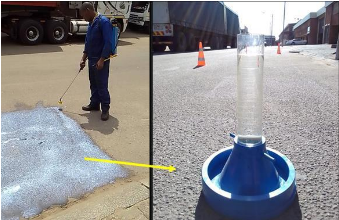
Figure 65: Labour-intensive application of a Nano-Silane Nano-Polymer (NSNP) clear-seal to provide a deep penetrating water-repellent surfacing to protect against the ingress of water into the pavement structure, preventing the formation of potholes (Photographs provided and published with permission [21])
