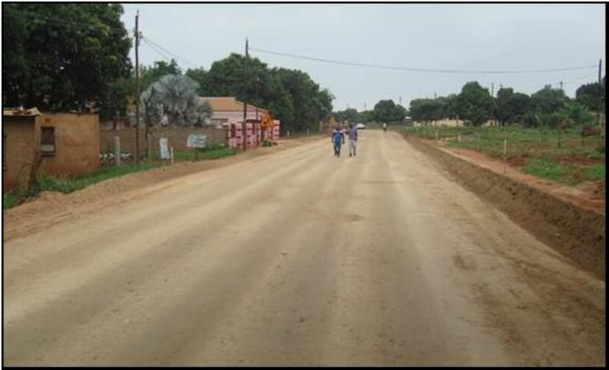
Figure 28: Recycled road with NME stabilisation opened to local traffic to provide access to houses – with no protective prime or surfacing added (note the same pink painted façade of the same house shown in Figure 24)
