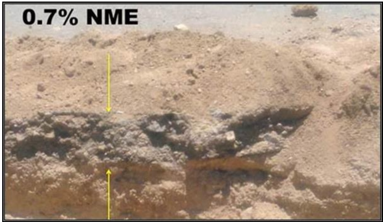
Figure 38: Cut through the stabilised sub-base constructed using a water-cart for distribution of the 0.7% anionic NME stabilising agent added to the construction water, mixed by grader and compacted
