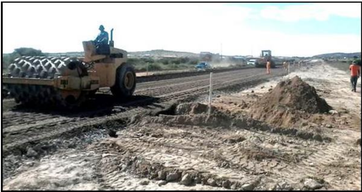
Figure 44: Compaction and cutting of final layer levels
