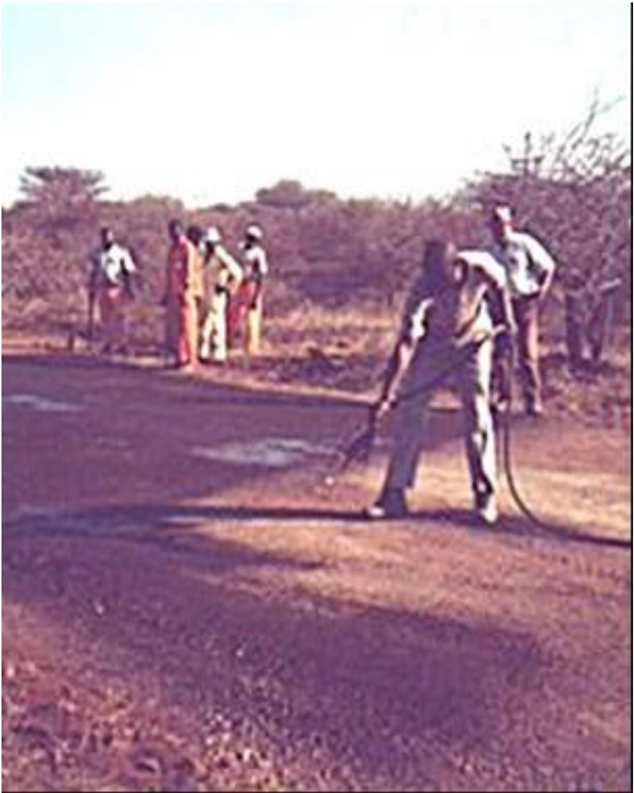
Figure 51: Application by hand of an enrichment layer
