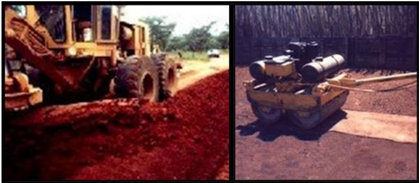
Figure 50: Mixings by grader and compaction using hand operating compaction equipment
