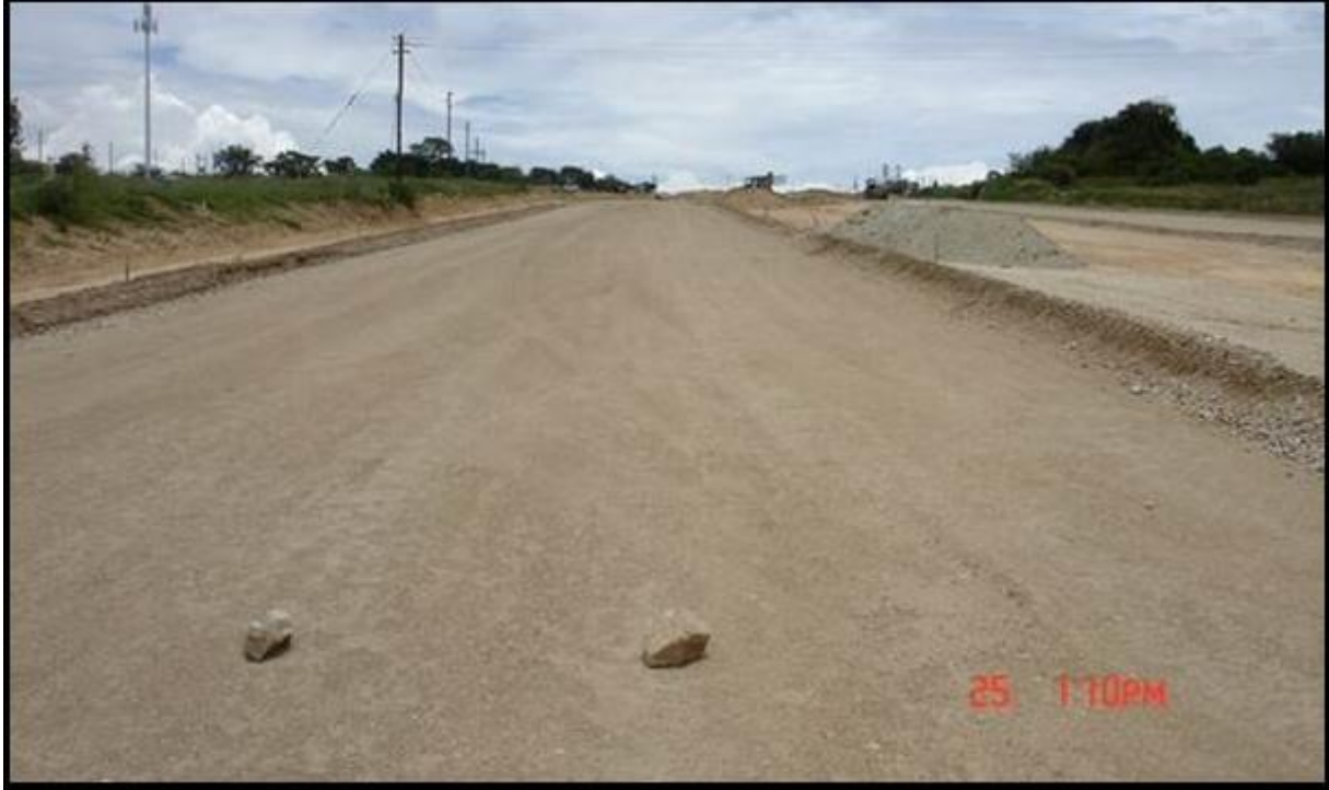
Figure 40: Condition of the sub-base after being subjected to the rain
