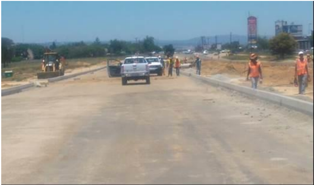
Figure 11: Prepared sub-base with installed curbs for the inter-city freeway under construction
