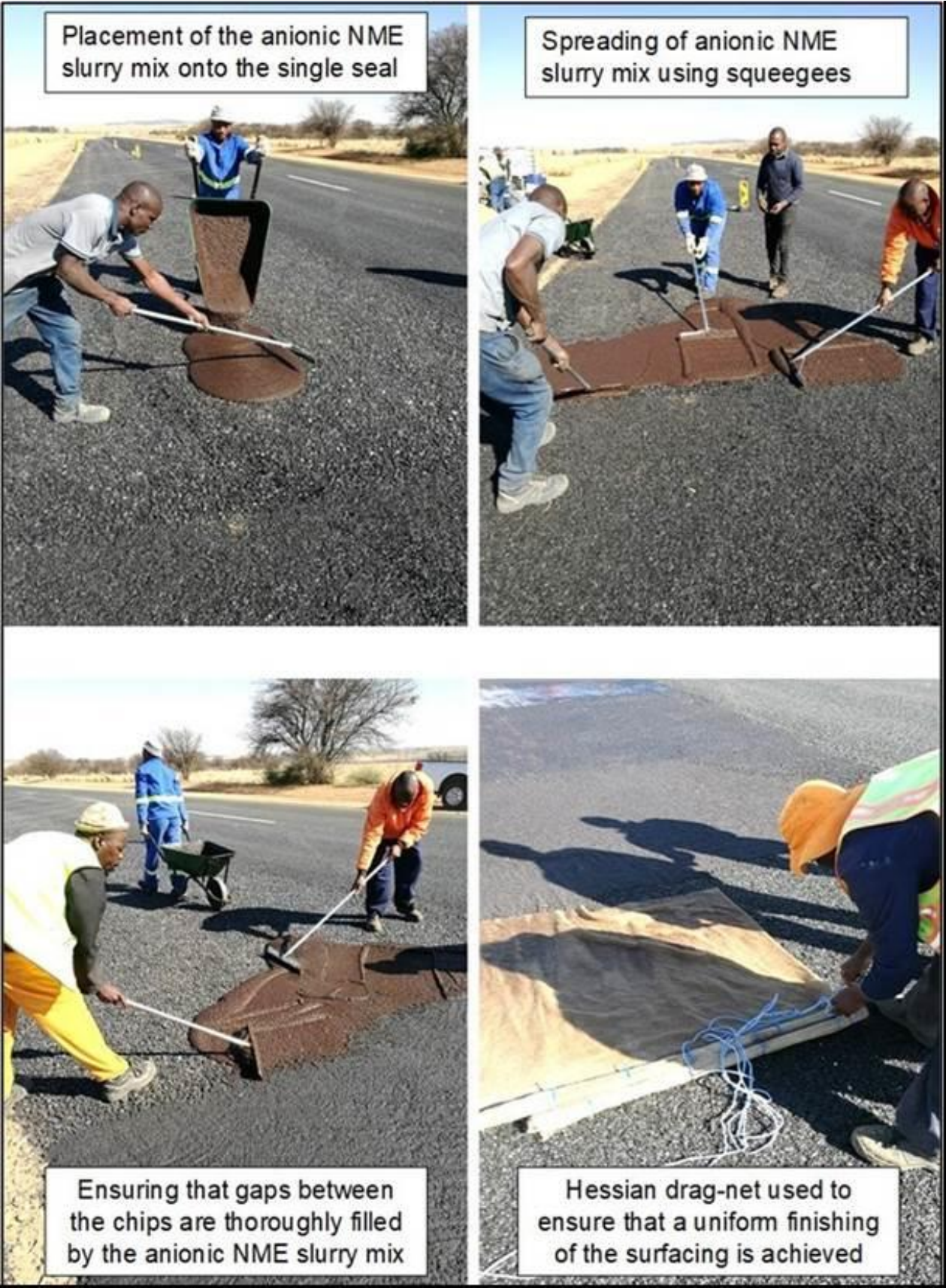
Figure 53: Labour-intensive construction of a modified Cape seal using an anionic NME binder with the slurry mixed on site next to the road
