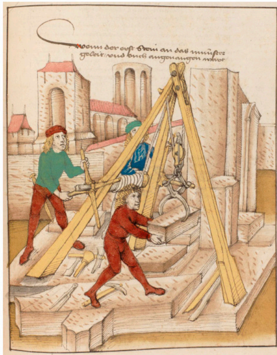
III. 1. Medieval builders use a tripod with blocks and tackles and with a winch to lift stone blocks. The picture is from a 15th century manuscript. To hold the stone block, a block tongs are used. With the help of the tripod, it is possible not only to lift a stone block but also to move (drag) it in the horizontal plane.
