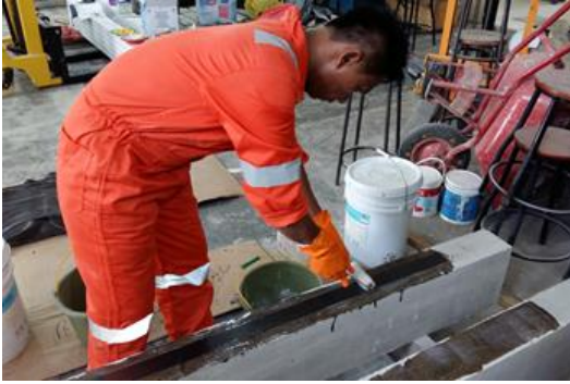
Figure 2. Installing the CFRP plate at the bottom of the beam
