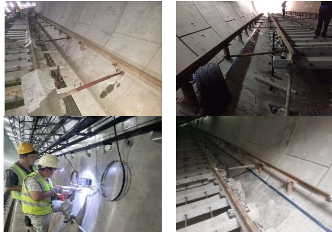
Figure 10. Construction photographs showing the optical fiber placement
