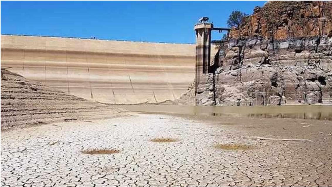
Figure 4. Gamka dam running dry 2009-2011, 2017-2019.
