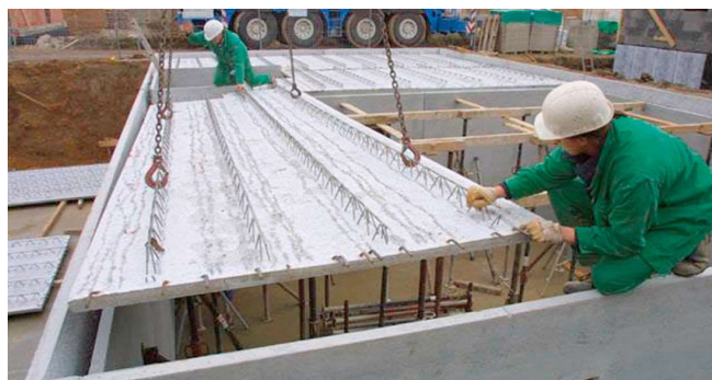
Figure 3. Filigree ceiling on the construction site [31].
