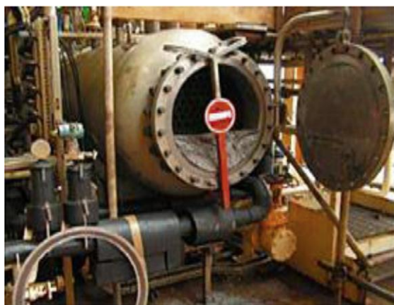
Figure 1: Pictorial view of ingress of fine sand into a production separator that resulted in production shut down (Oyeneyin, 2015)
