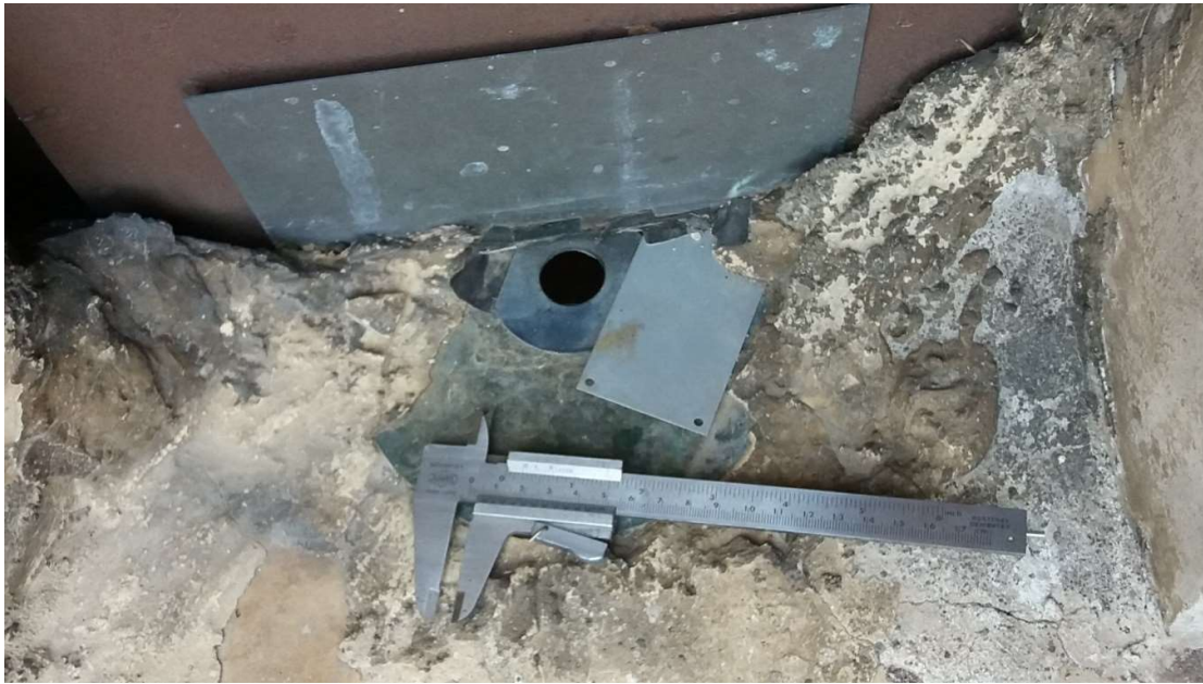
Figure 1. The pinhole of the meridian line, as seen from the outside of the Basilica. The North is here up right. This external area of brick and cement determines the air turbulence of the solar image.
