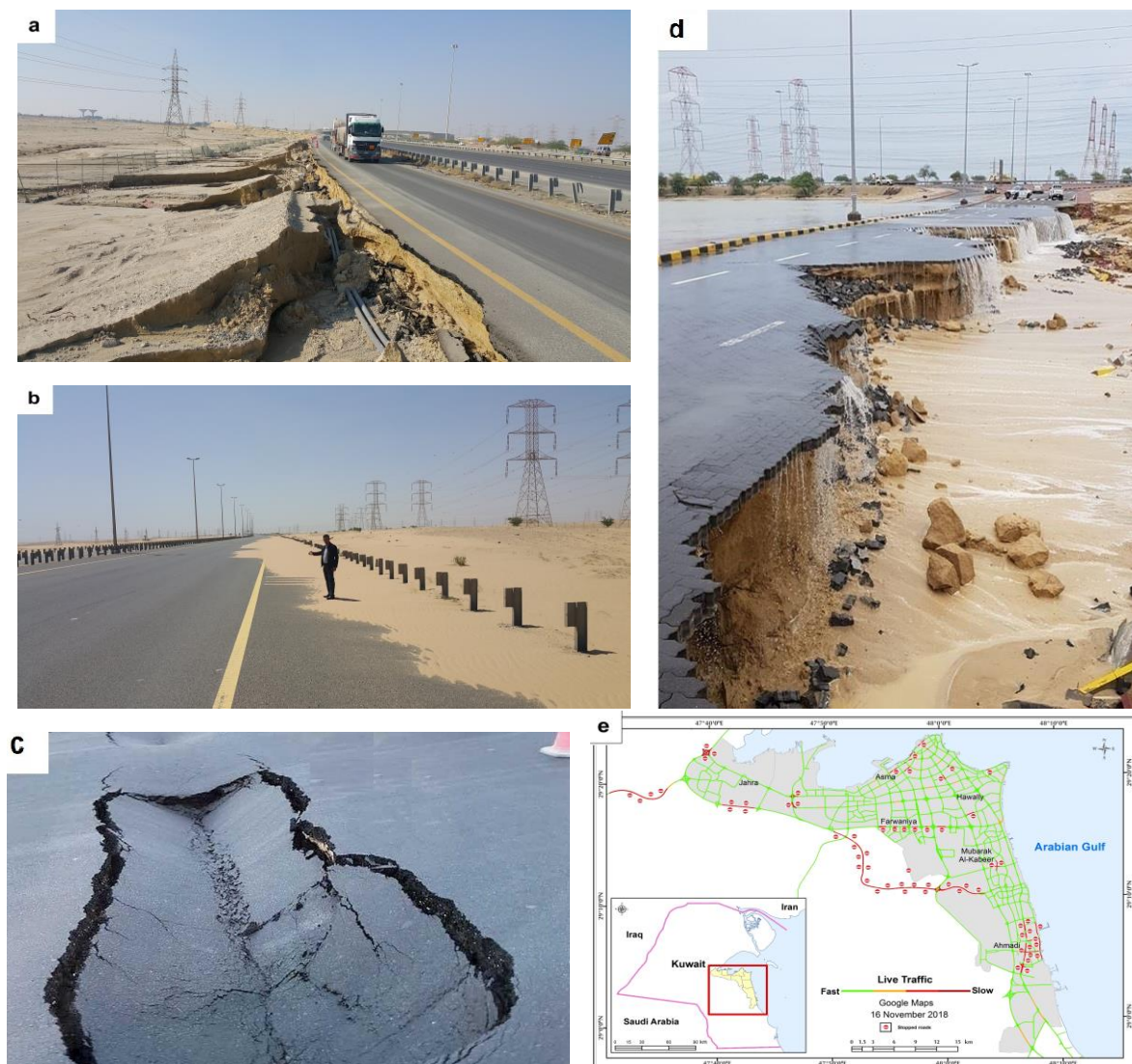
Figure 6. Some natural hazards in Kuwait. A) Impact of flash flood on road 40 on 17 November 2018. B) Sand movement on Al Subiya Road, in March 2018. C) A sinkhole or A collapse on the 6th Ring Road. D) Impact of flash flood on roads and infrastructure on 15 November 2018. E) Roads stopped/closed after a rainstorm, Source: Live traffic, google maps, 16 November 2018.
