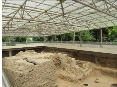
Figure 10. Truss roof, near the Syntagma square in Athens, Greece [10]
