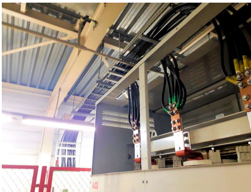
Figure 1. Multi-strand cable line in a car factory. Source: own work, A. Cywiński.
