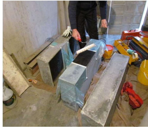
Figure 6. Apply of the CFRP plates on B-1 and B-2 deep beam.
