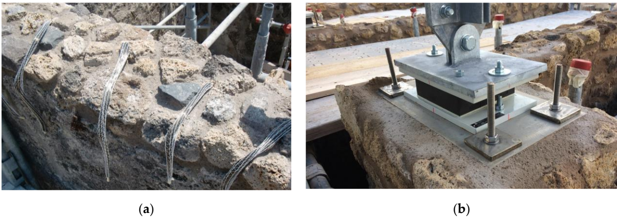
Figure 11. (a) Basalt fibre ropes in the masonry top wall. (b) The rubber support device.
