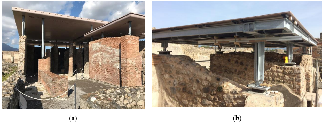
Figure 6. The new roof in the Championnet area: (a) a view of the new roof; (b) Steel structures before coating
