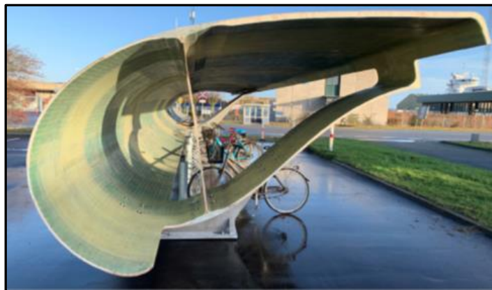
Figure 7. Examples for rotor blade repurposing: bike shed (source: Re-Wind and Port of Aalborg, Denmark, Wind Europe Report 2020), reproduced with permission of WindEurope [13].
