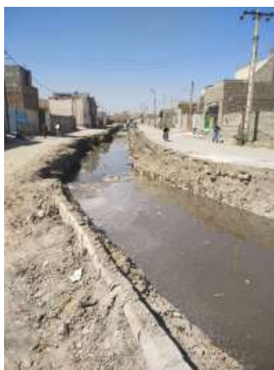
Figure 5. Joining small streams of sewage and pouring them into larger canals
