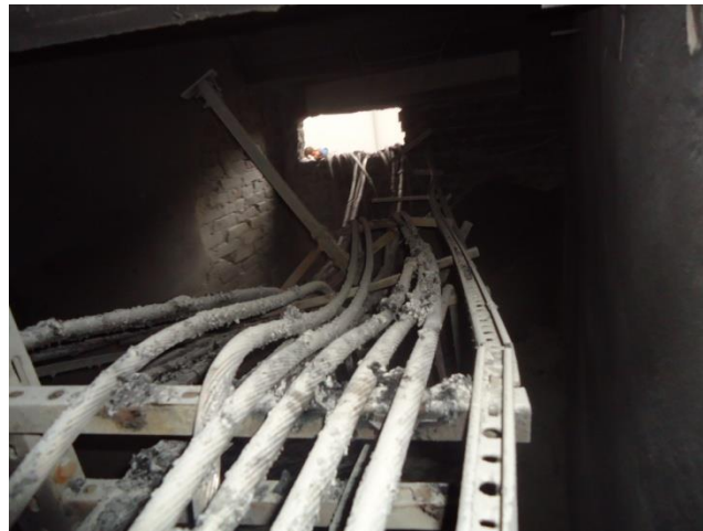
Figure 1. A destroyed cable supply system [16]
