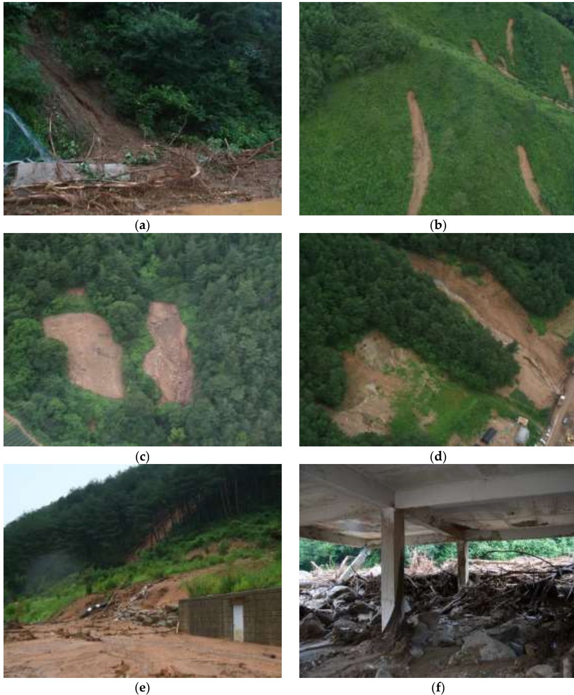
Figure 3. (a)– (e): observed landslides and f) debris deposit.
