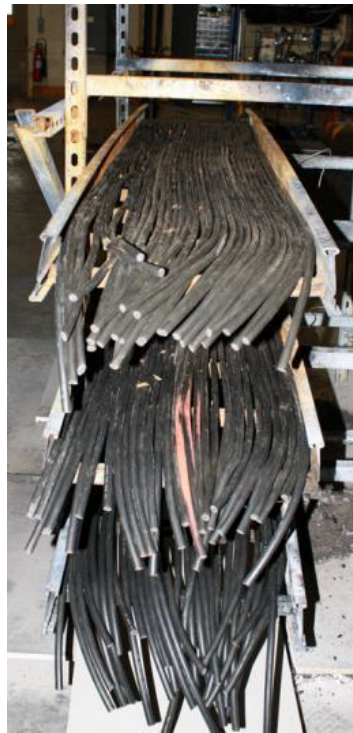
Figure 3. Photograph of the cable arrangement in MT3, taken from the CHRISTIFIRE report [15].
