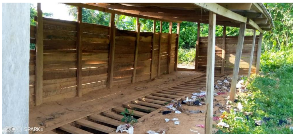
Fig. 7. An open public pit latrine
