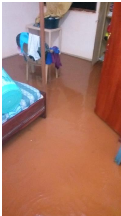
Fig. 6. A flooded bedroom after a heavy downpour
