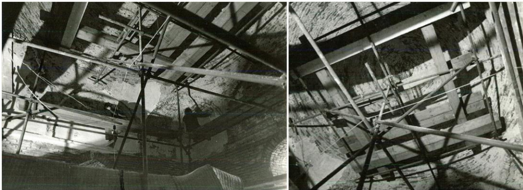
Figure 12. Repair of ceiling plaster under the dome. (author).
