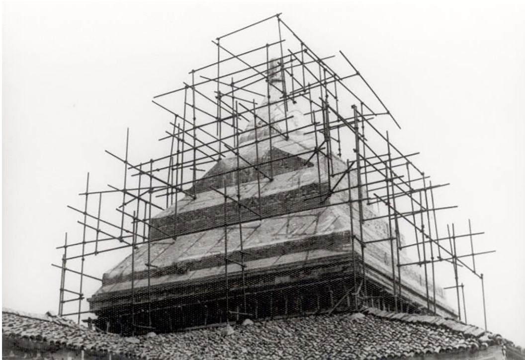
Figure 13. Complete substitution of tiles on dome's exterior. (author).
