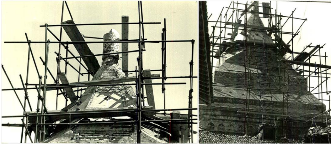
Figure 11. Renovation of the tiles on dome's exterior. (author).
