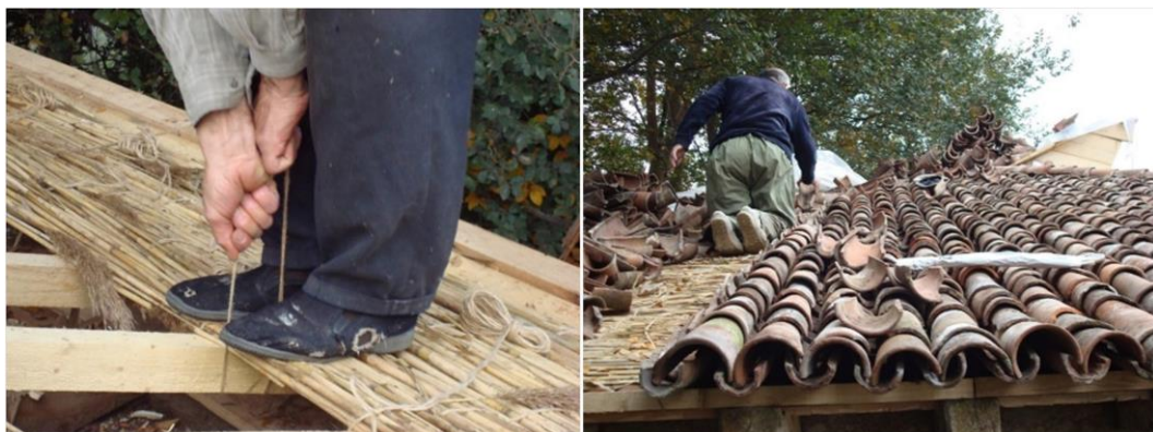
Figure 14. Replacement of the straws and clay roof-covering. (author).
