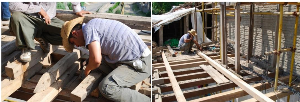
Figure 15. Renovation process of wooden structure of the roof (author).
