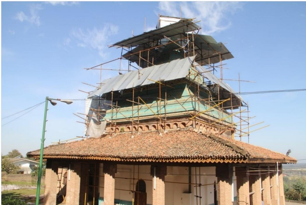
Figure 17. Reassembling dome's tiles. (author).
