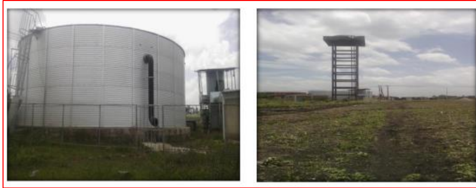
Figure 3: service and elevated tank
