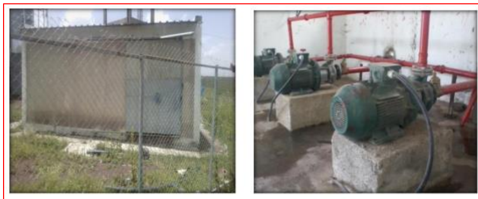
Figure 4: Pump house and pumps
