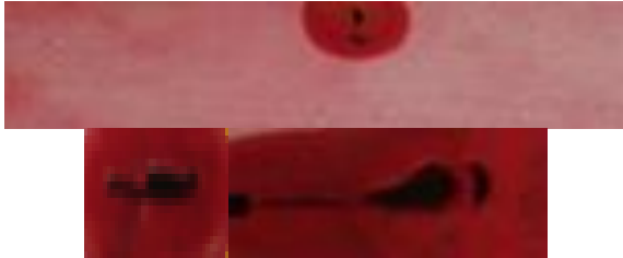
Fig. 5: the defects that traced with PT test
