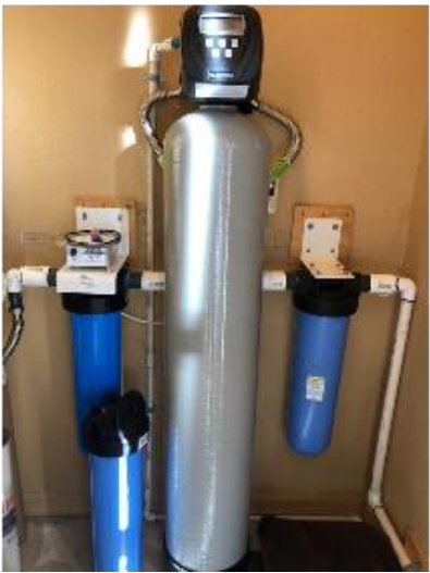
Figure 12. From right to left: sediment filter, charcoal regeneration, ultraviolet filter (spare tank in front)
