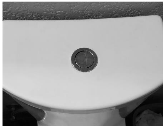
Figure 15. Low flow (dual flush) toilet, installed
