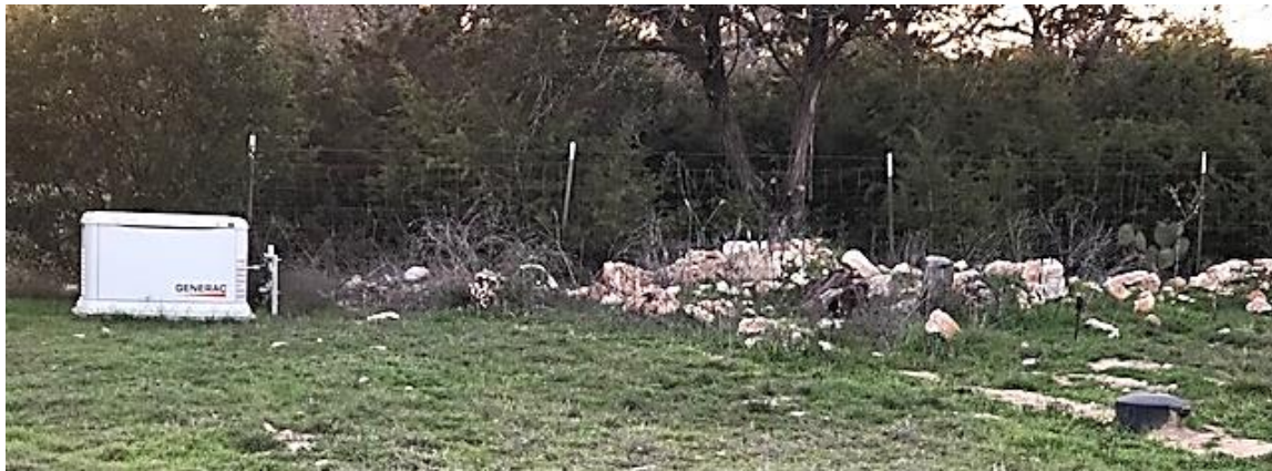
Figure 23. Generac 22 kWh whole-house generator and propane tank
