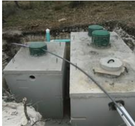
Figure 16. Biological Accelerated Treatment plant during installation
