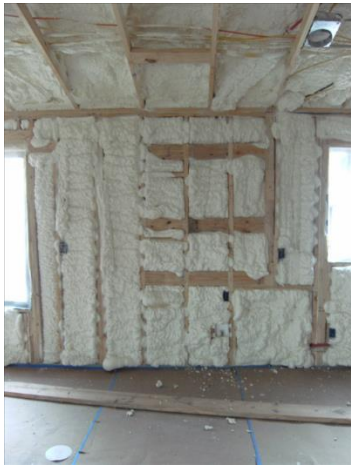
Figure 5. Open-cell spray-foam insulation
