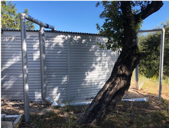
Figure 8. First flush system
