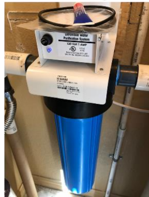
Figure 13. Ultraviolet purification and example light
