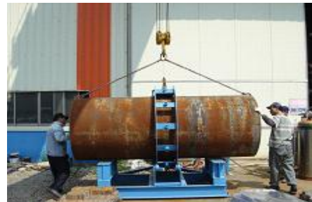
(b) Installation of Steel Tube (Specimen)
