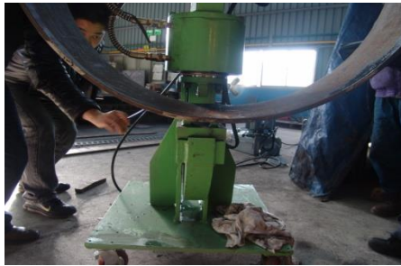
(a) Installation of C-TYPE JIG
