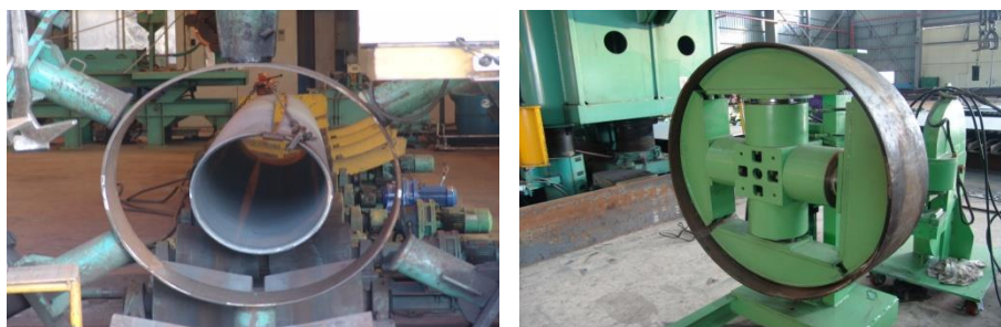
(a) Partial deforming of steel tube (b) Installation of tube expander
