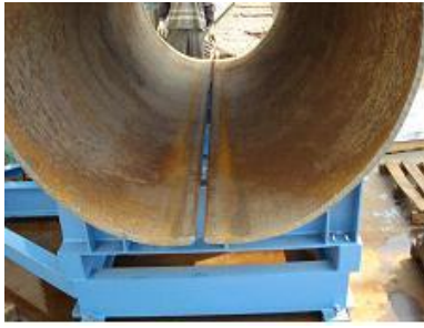
(a) Rupture of Temporary Joints(about 500°C)
