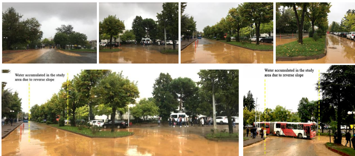
Figure 3. Collection of rainwater in study area due to inverse slope
