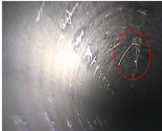
Figure 8. Root penetration into the distribution pipe during subsurface cleaning in June 2016.
