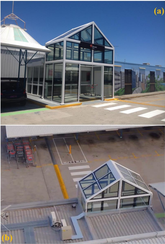
Figure 1. Entrance porch (atrium) of Warwick Grove Shopping Centre in Warwick (Perth, WA, Australia) constructed using 18 solar windows supplied by Clearvue Technologies Ltd. (Perth, WA, Australia). (a) front view and (b) top view.
