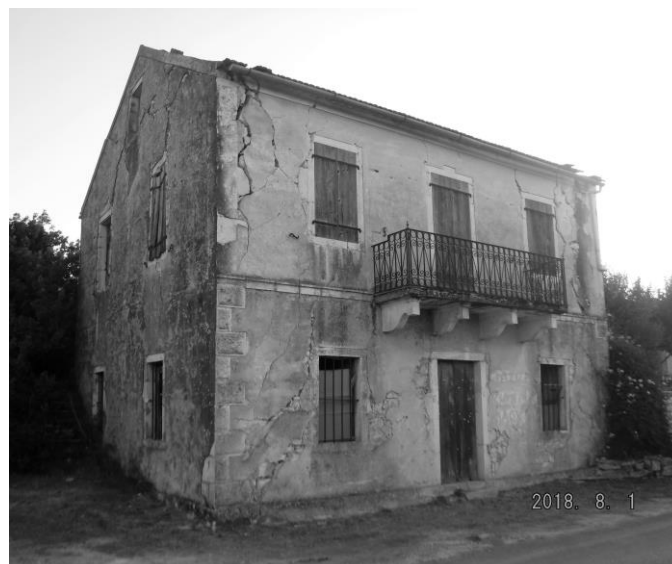
Figure 3. Two-storey house built before the 1953 earthquake near Fiskardo, in present condition.
