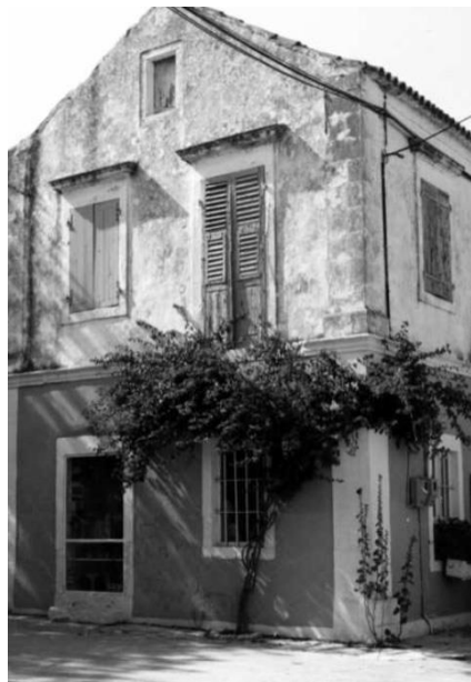
Figure 2. Two-storey house before 1953 earthquake, in [11] (p.12).
