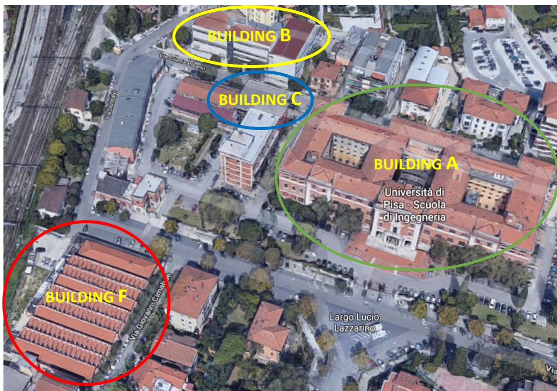
Figure 1. A complete view of the buildings of the School of Engineering (University of Pisa).
