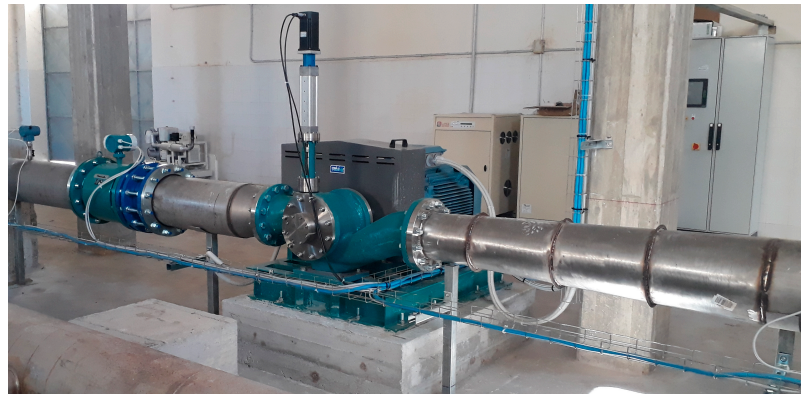
Figure 6. PRS turbine prototype installed in the study case.
