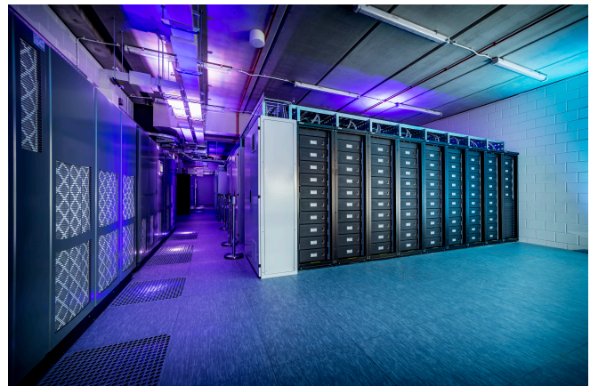
Figure 2. Racks with part of the 2.8MWh energy storage system at the “Johan Cruyff Arena”. [Photo courtesy of Eaton].
