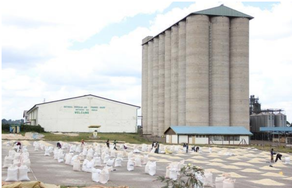
Figure 4. Maize drying, packaging and storage at the national cereals and produce board of Kenya (source: https://www.nation.co.ke/oped/opinion/africa-economy-growth-government-development-youth/ ). Similar storage structures exist at The Tanzanian National Reserve Food Agency.
