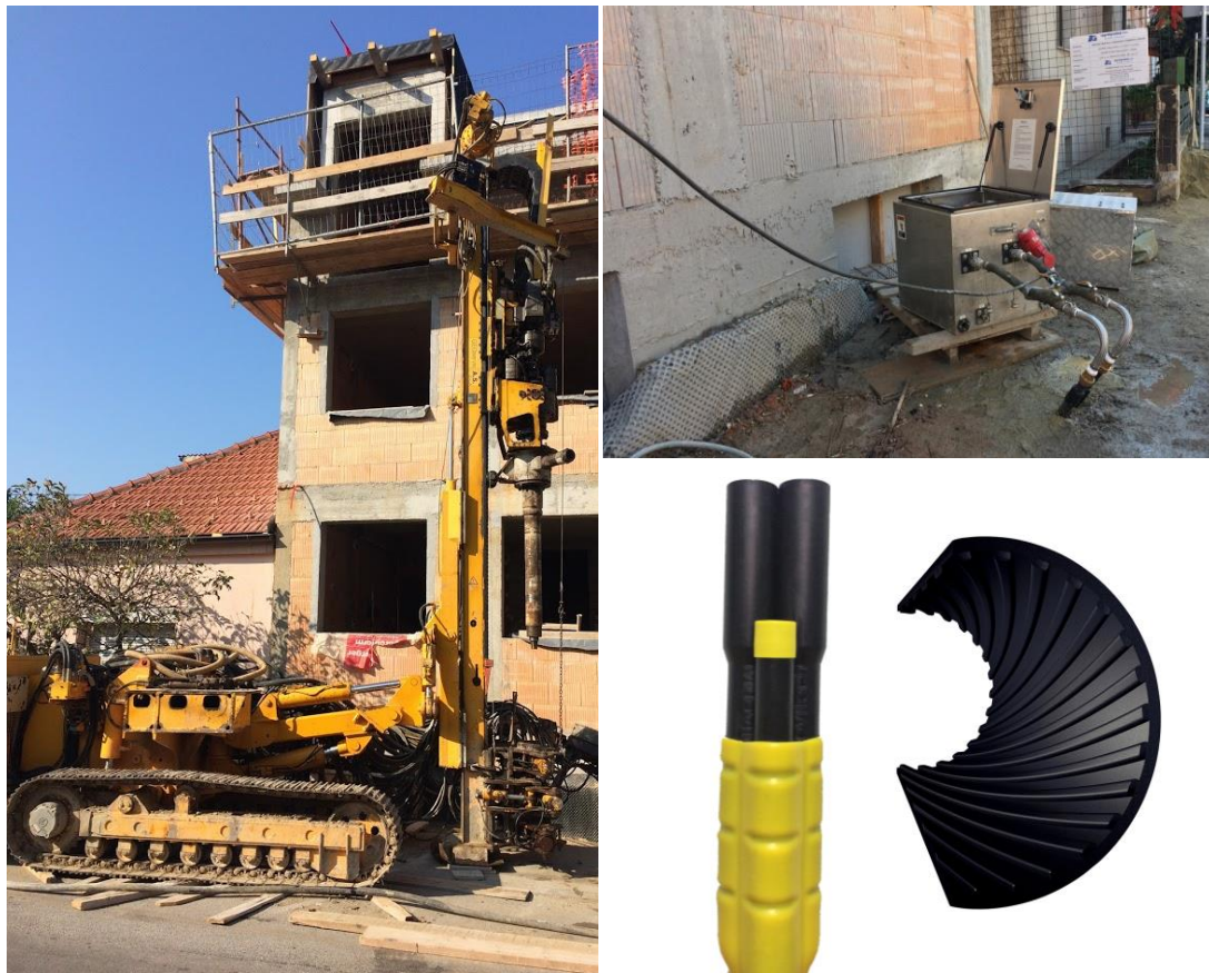
Figure 3. a) Drilling of the BHEs b) performing the thermal response test c) TurboCollector™ pipe
