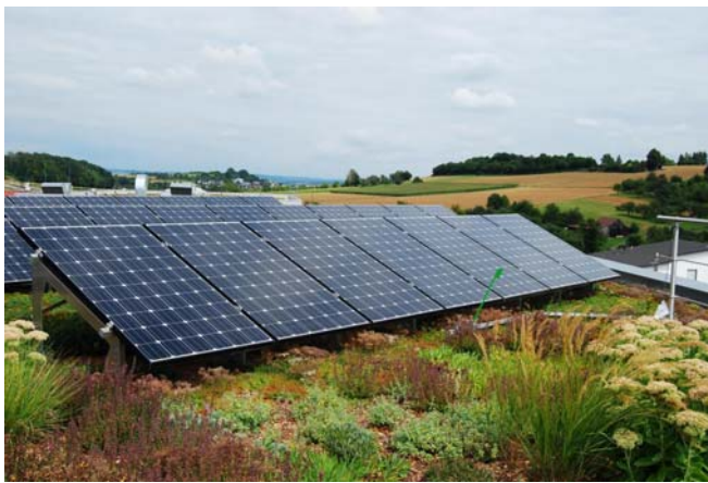
Figure 1. The green roof provides a superimposed load. There is no roof penetration thanks to the superimposed load principle. [Photo courtesy of ZinCo].
