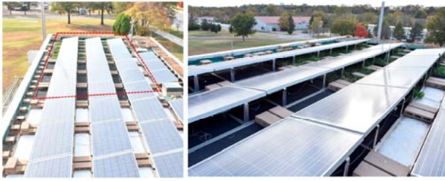
Figure 10. The PV modules tested during one solar year installed on bituminous membrane and on a green roof. The tilt angle for all the modules was fixed at 10° facing south. [Reproduced from Ref.24, with kind permission].
