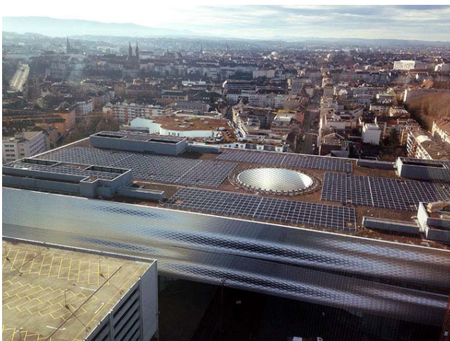
Figure 4. The 1189.1 kW solar green roof on main exhibition hall of the new Messe Basel. [Photo courtesy of Tritec Project Engineering].
