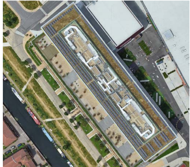
Figure 12. The four-storey London Olympics International Broadcast Centre hosts a 2,500 m 2 green solar roof whose habitat attempts to mimic the open habitat of the Thames river corridor. [Photographs from Google Earth].
