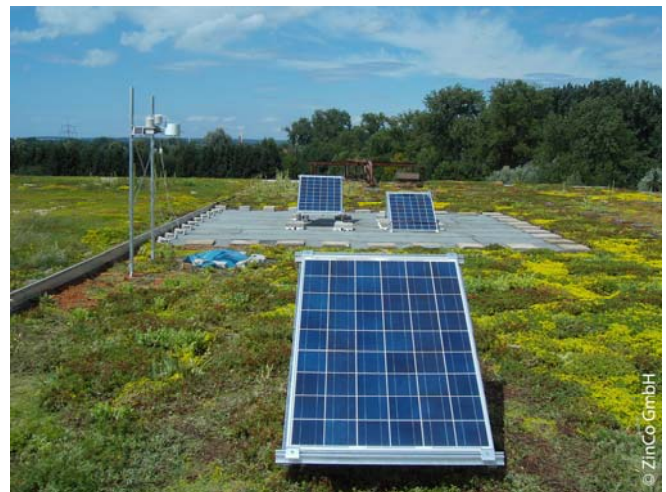
Figure 9. The PV modules tested during one solar year installed on bituminous membrane and on a green roof. [Photo courtesy of ZinCo].
