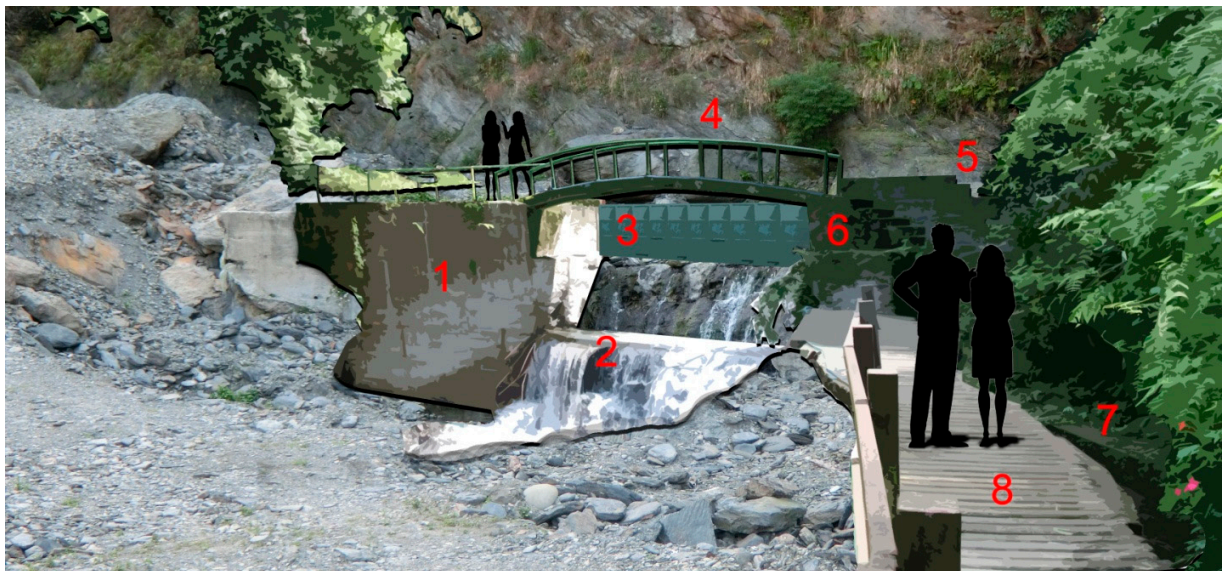
Fig. 6. Reconstruction of the diversion weir according to the old imagery. 1-the main body of the weir, 2-deflector, 3-original spillway gates, 4-Green bridge, 5-access stairs, 6-bridge stairs, 7-supply channel, 8-old plank path. (Source - Author)
