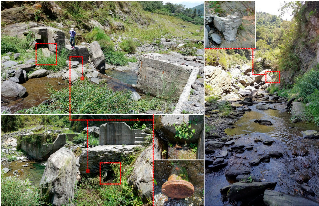
Fig. 7. Details of the intake weir showing the position of inflow and desilting openings on left. On right there is Shanping creek riverbed in front of the intake weir indicating the remains of the Lovers bridge. (Source - Author)
