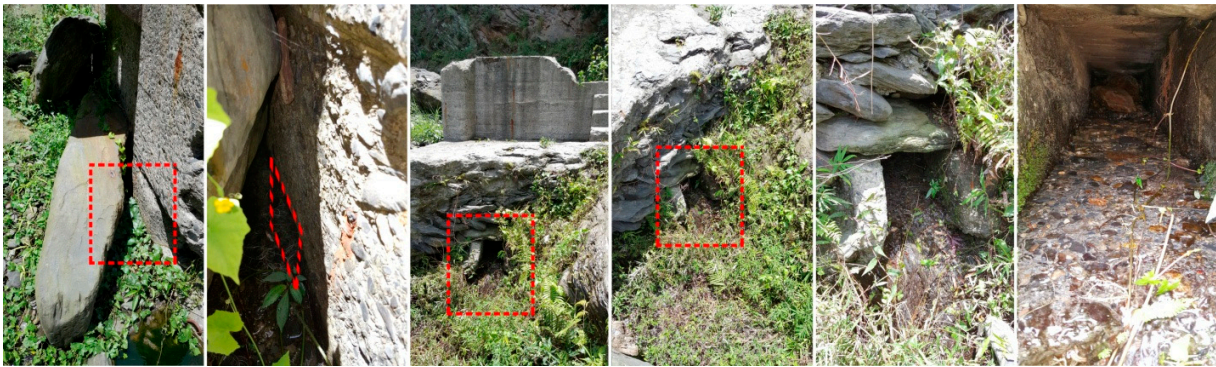
Fig. 8. Inflow opening is located behind a rock and is blocked with alluvial sand and rocks. On the other side of the dam the opening is clearly visible (Source - Author)
