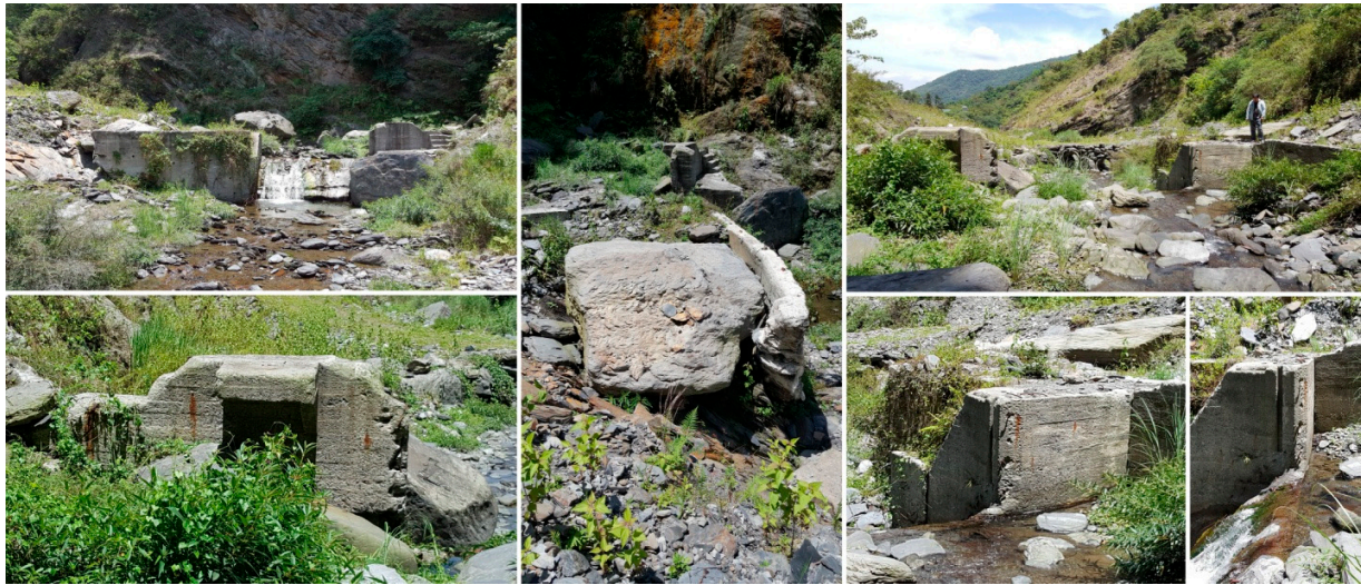
Fig. 5. Remains of the water intake weir show clearly shift of the dam body due to giant rocks from a landslide. (Source - Author)
