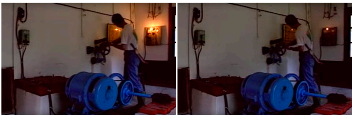
Fig. 14. [13] Interior of the Shanping hydropower plant including three phase self-excited generator powered by triple V-belt transmitting torque from turbine shaft with flywheel connected to the horizontal Francis turbine behind the wall.
